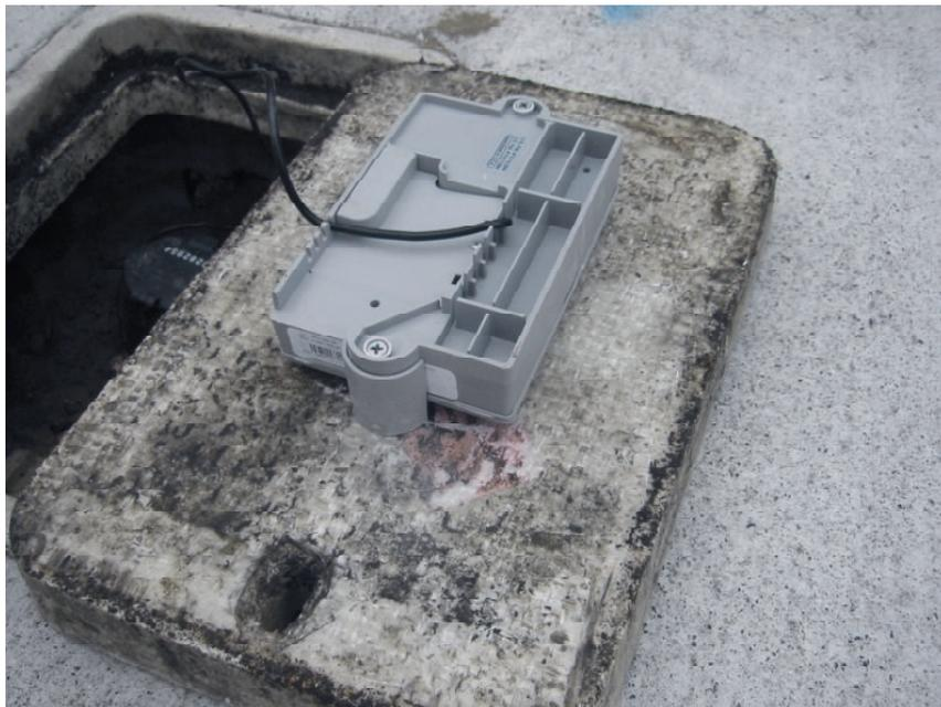
Top: Water meter with transducer.
