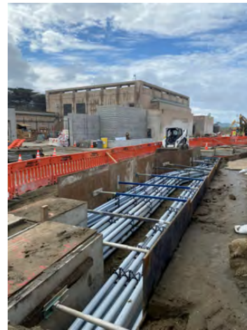
New underground conduit raceway installation at Great Highway in May 2023
