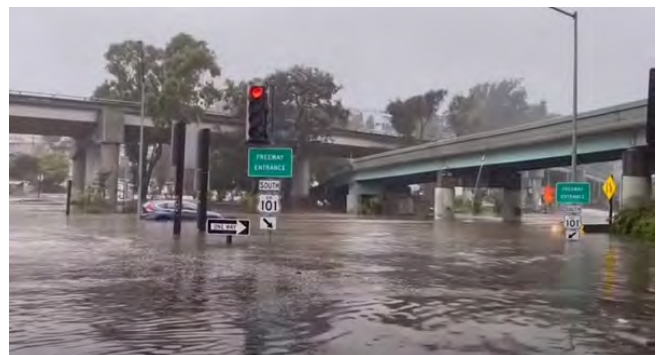
Flooding at the I-280/Hwy 101 interchange at Lower Alemany area, during the rainfall of January 2023
