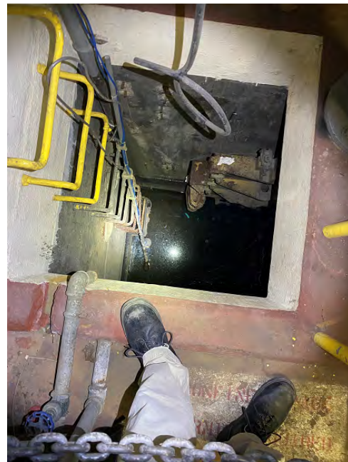
Entrance to Geary Underpass Pump Station
