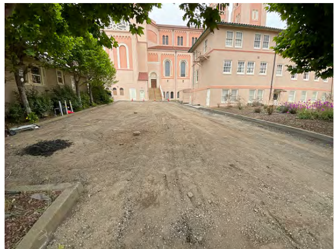
Excavation work begins at St Anne of the Sunset.
