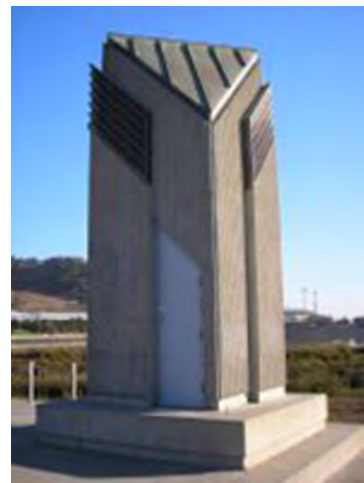
Air Vent for the Underground Sunnydale Pump Station.
