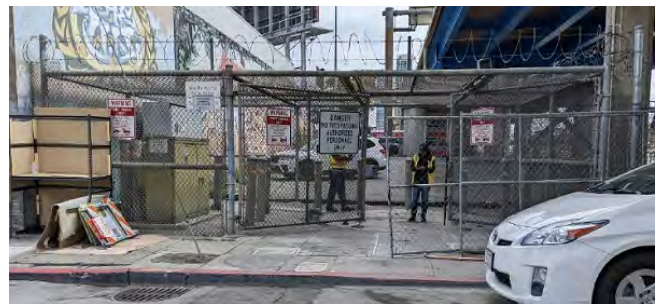
Merlin Morris Pump Station - Existing Fencing Enclosure to be Upgraded.
