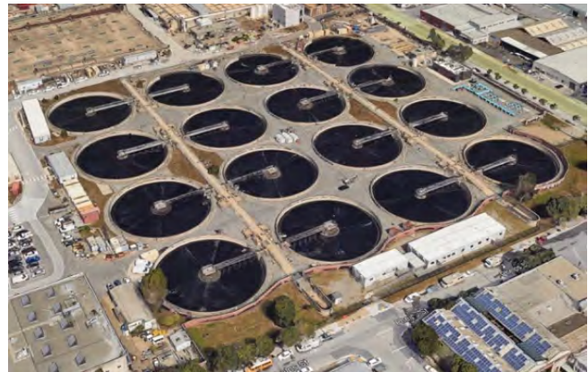
Aerial Photo of Secondary Clarifiers at SEP
