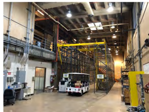
Inside of Bldg SEP 940
