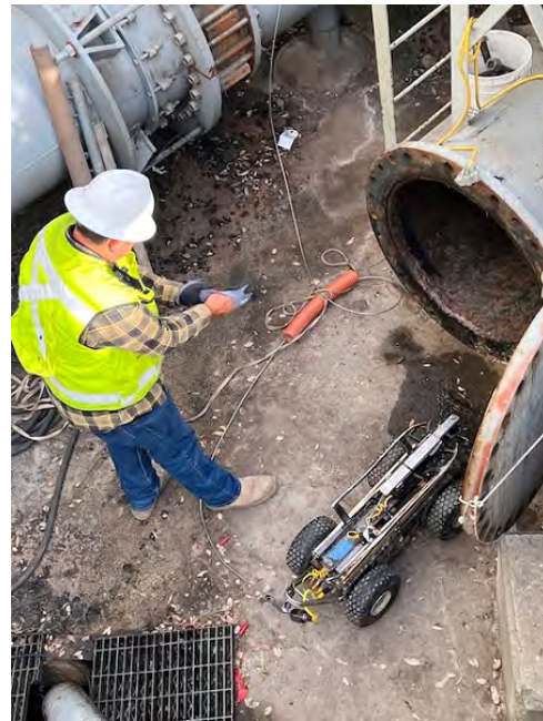
Interior CCTV camera inspection of the discharge manifold
