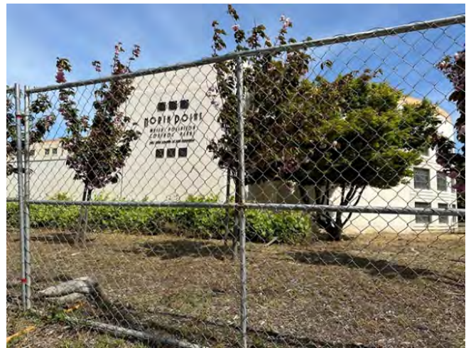
Temporary Chain link fence at North Point Facility
