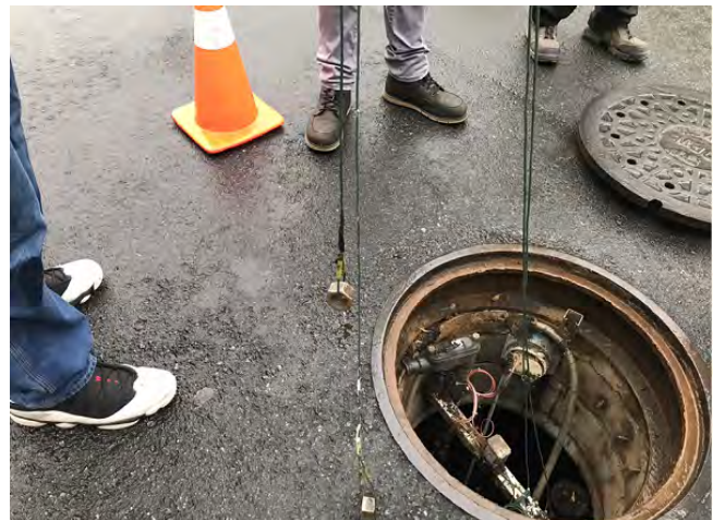
Project team performing field measurements and investigation.
