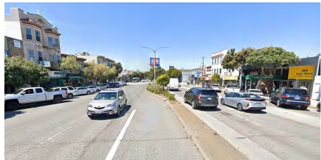
A portion of Geary Boulevard between 19th and 20th Avenue which is a critical part of the project corridor
