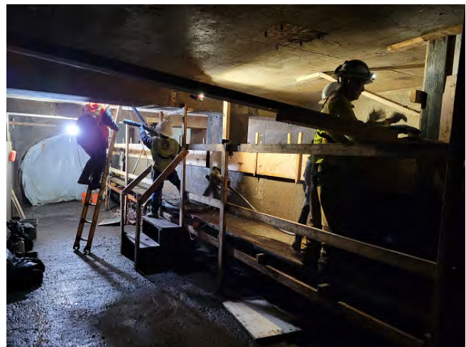
Rebuilding the Concrete Weir.
