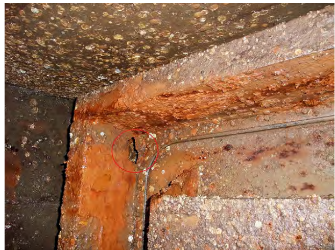
Brannan CSD Existing Damaged Butterfly Discharge Valve.
