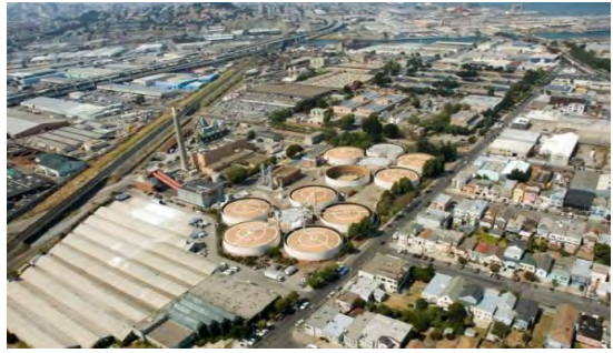
Southeast Treatment Plant
