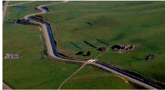
South Bay Aqueduct
