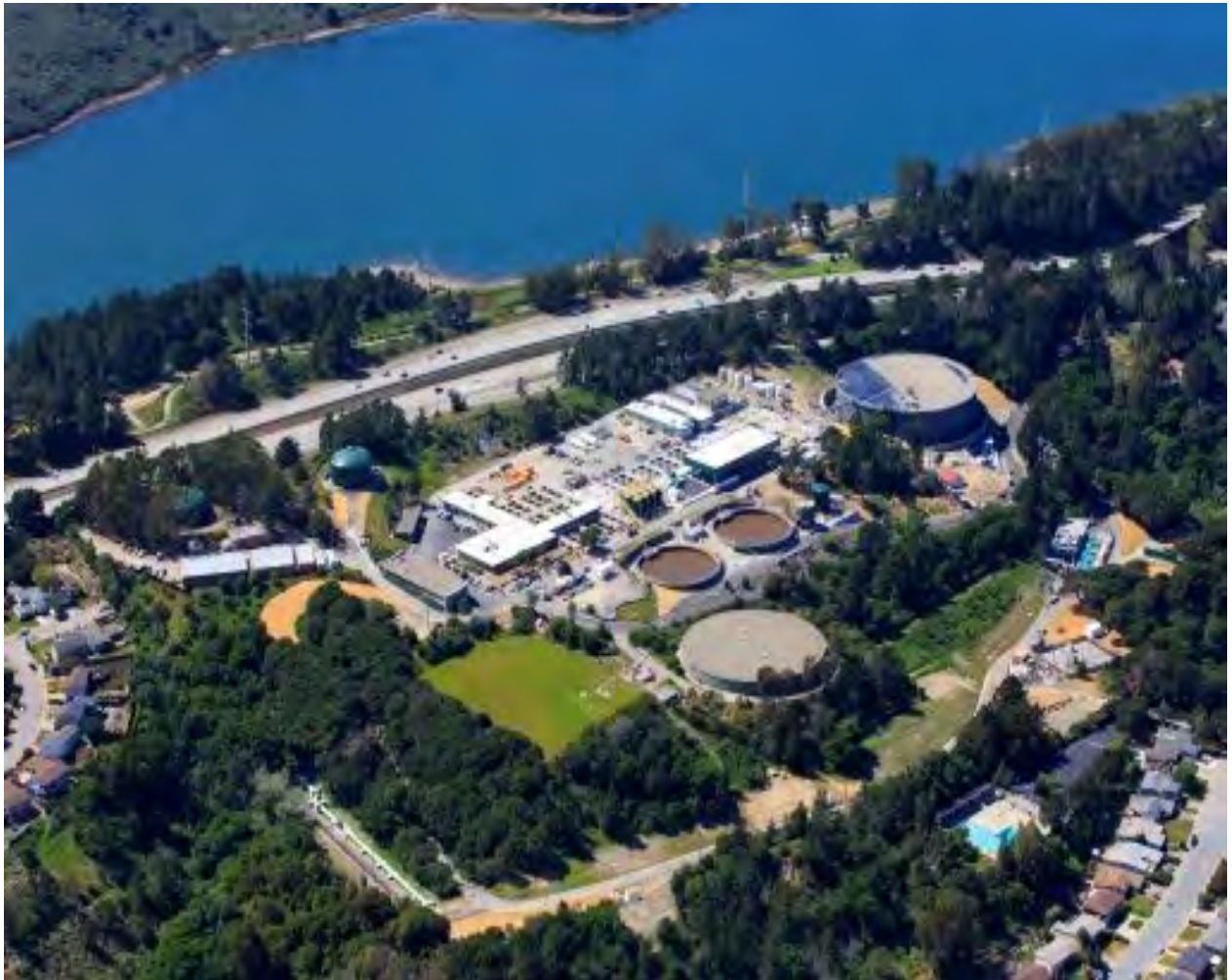
Photo: Harry Tracy Water Treatment Plant, April 2015
