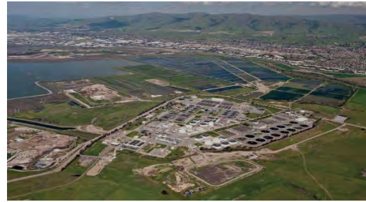
San Jose-Santa Clara Regional Wastewater Facility
