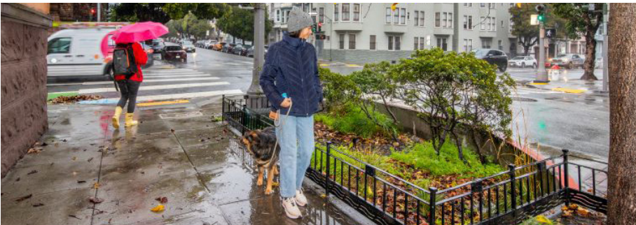
Wiggle Neighborhood Green Corridor Rain Gardens - Hinahawakan ng Wiggle Neighborhood Green Corridor project ang 1.2 milyong galon ng tubig-ulan kada taon. Lokasyon ng larawan: Fell Street at Broderick Street.
