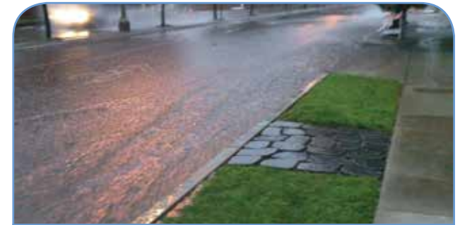
The street profile is designed in part to convey stormwater to collection points, such as bioretention planters and catch basins. Changes to the street profile can cause inadvertent and detrimental impacts related to runoff and flooding.
