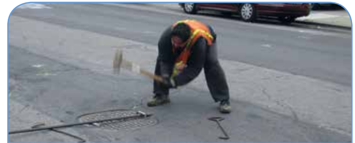
Clear space around water valves is necessary to access, operate, and maintain the valves.
