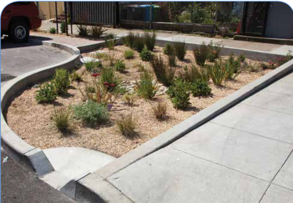
Typical Green Stormwater Infrastructure bioretention planter
