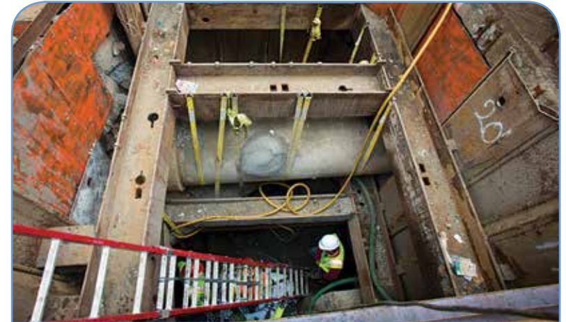
Maintaining minimum clear spaces around existing underground SFPUC assets ensures that SFPUC crews and contractors are able to excavate around those assets and install shoring for required maintenance work.
