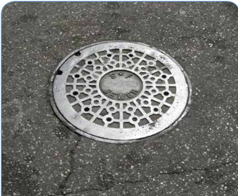
A solid, paved working surface is necessary around manholes to facilitate maintenance work.
