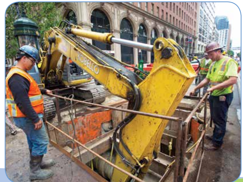
Maintaining minimum clear spaces around existing underground SFPUC assets ensures that SFPUC crews and contractors are able to excavate around those assets and install shoring for required maintenance work.
