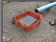
Protect all existing drains and newly installed drains. See Figure 4.12
