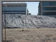
Excess soils are stockpiled and covered for dust control. See Section 5.5
