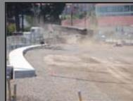
Apply water or stabilizers to minimize dust. See Section 3.5
