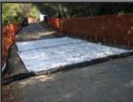
Install to minimize tracking of soil and sediment. See Section 3.1
