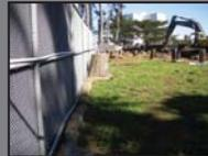
Attach silt fence to construction fencing to screen project and provide wind protection. See Section 4.14
