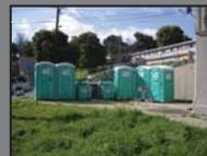
Properly locate sanitary facilities to prevent discharge to storm systems. See Section 5.6
