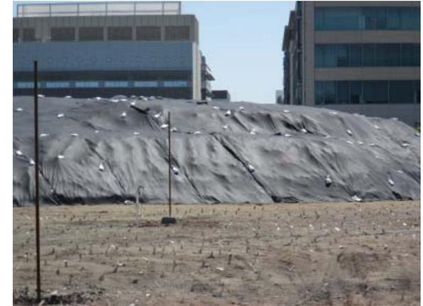
A properly protected stockpile with a plastic cover anchored down by gravel bags.
