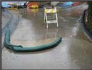
Install to reduce runoff velocity and to collect sediment. See Section 4.11
