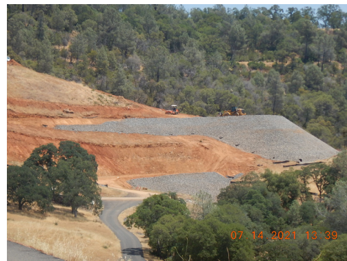
Priest Spoils Disposal Site Development underway
