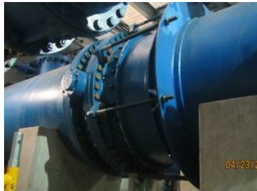
Picture of TUV101 66" BFV @Tesla Valve House TUV101 Valve Replacement
