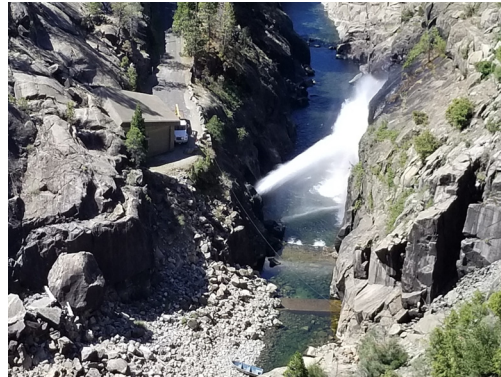
Discharge from the Instream Flow Release Valve
