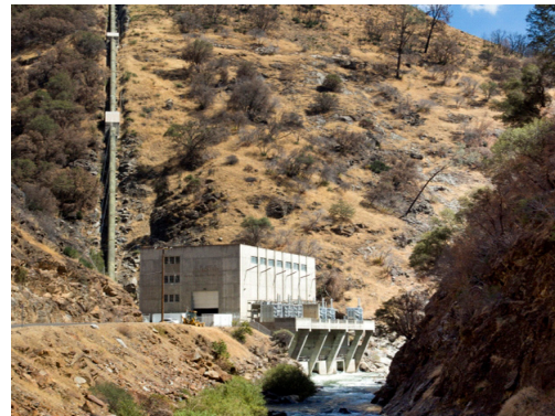
Generator Shaft at Moccasin Powerhouse
