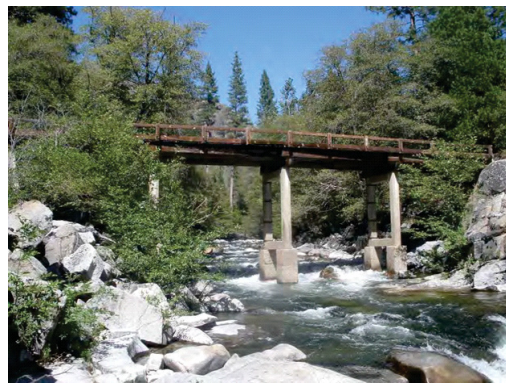
O'Shaughnessy Adit Access Bridge
