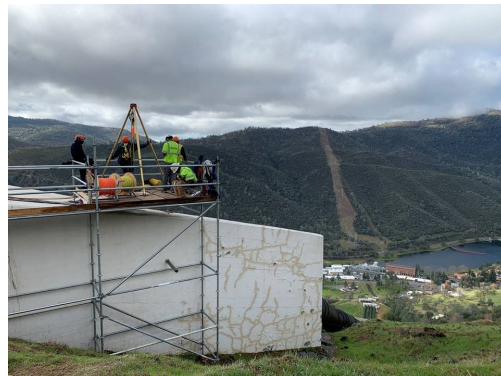
Moccasin Penstock – JOC field support for internal inspection
