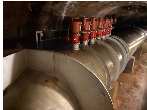
Diversion Pipe at O' Shaughnessy Dam
