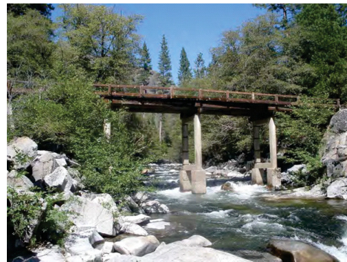
O'Shaughnessy Adit Access Bridge
