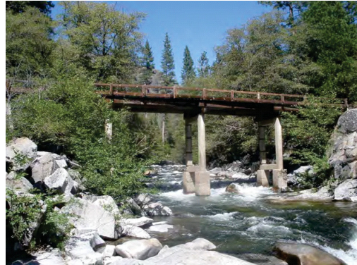
O'Shaughnessy Adit Access Bridge
