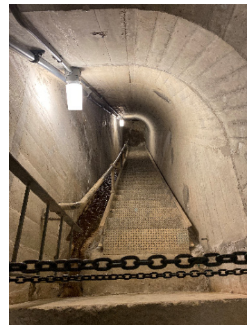
Inclined Stairway OSH Dam
