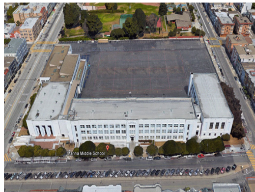
Marina Middle School Solar Project
