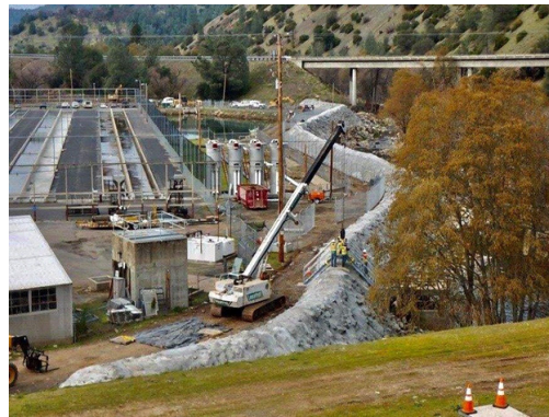
Construction of the flood control berm
