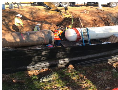
SJPL#1 – installation of a removable spool piece at Oakdale Portal
