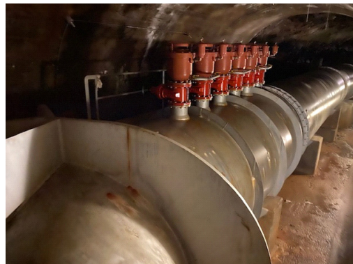
Diversion Pipe at O' Shaughnessy Dam
