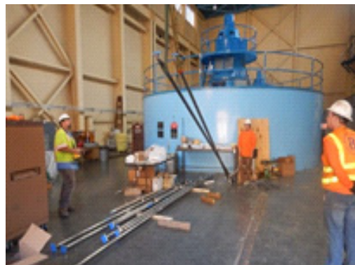
Workers using the overhead crane when accepting a delivery of equipment
