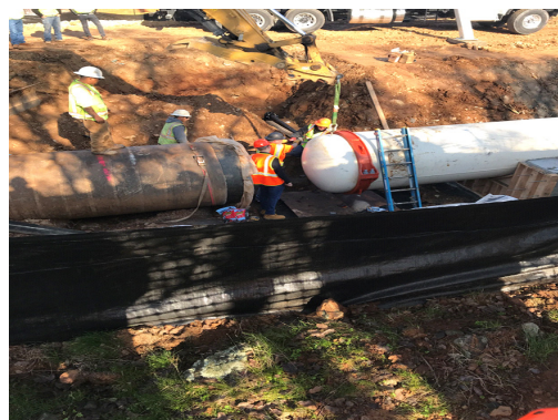
SJPL#1 – installation of a removable spool piece at Oakdale Portal
