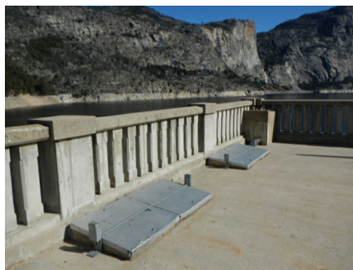
Bulkhead Slots Gates D & E – O' Shaughnessy Dam
