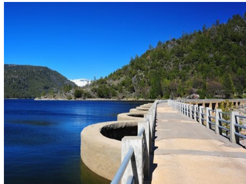
Lake Eleanor Dam Bridge
