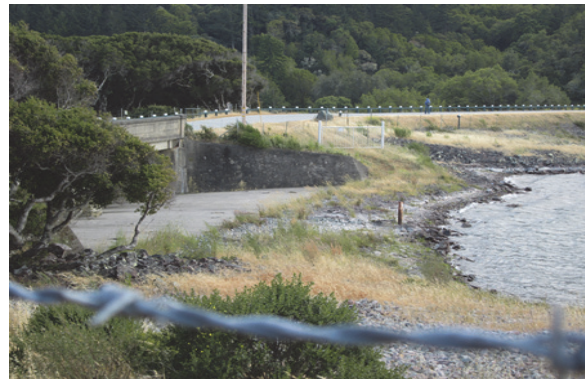
San Andreas Dam and Spillway
