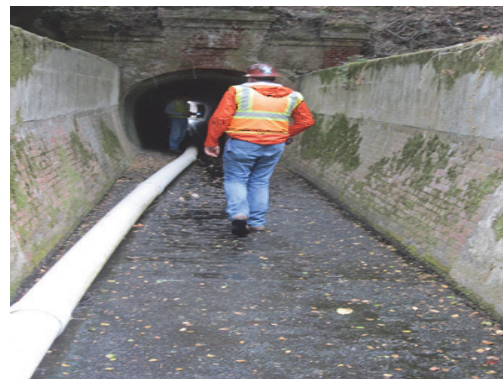
Pilarcitos spillway inspection
