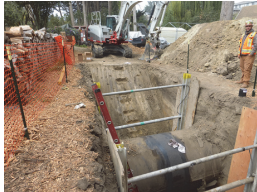
Exploratory Excavation for Corrosion Investigation
