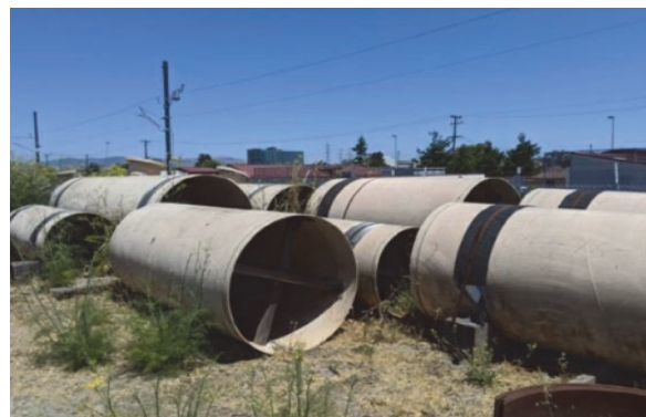
Stockpiled pipe segments to be used for repairs
