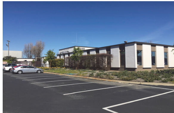
View of rear parking lot where lights and cameras will be added
