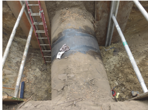
Excavated pipe for corrosion assessment
