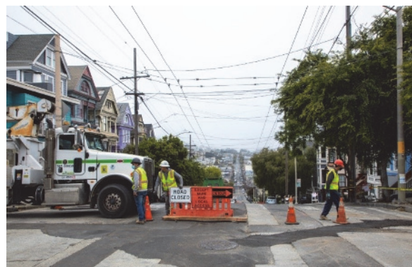
Water Main Replacement at Castro and 21st Street
