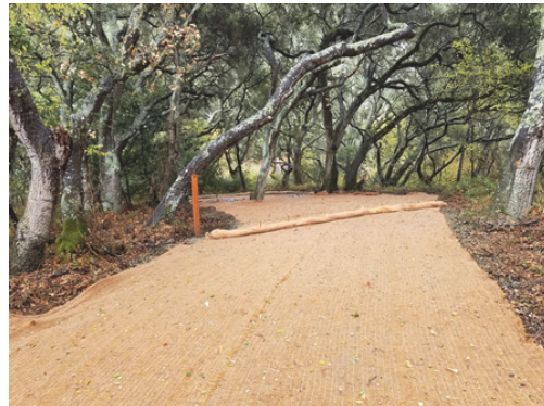
Site restoration work at Segment 1
