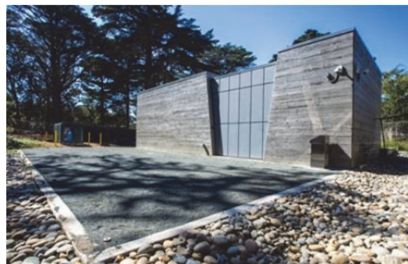
North Lake Well Station
