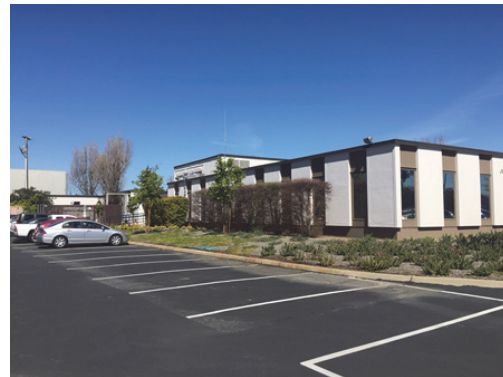
View of rear parking lot where lights and cameras will be added
