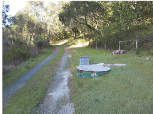
Corrosion Investigation Site in Hillsborough
