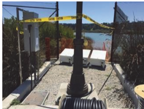
Aeration Mixing System Installation at Lake Merced Pump Station
