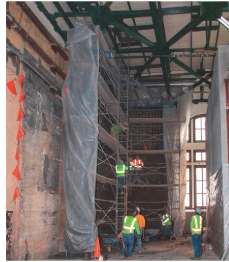
Roof installation of Pump Station No. 2
