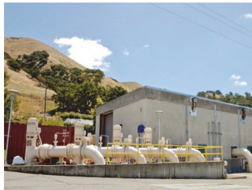
San Antonio Pump Station building looking southeast
