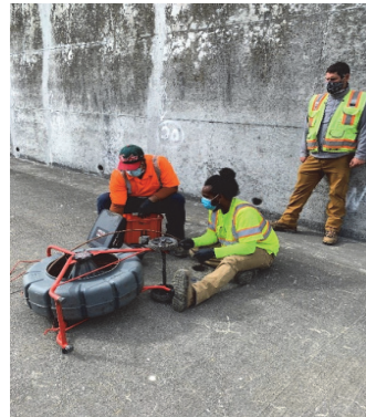
Sub-Drain Inspection at the Turner Dam Spillway
