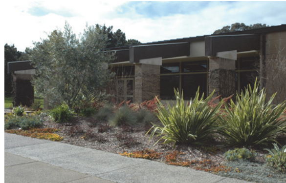
Existing Administration Building
