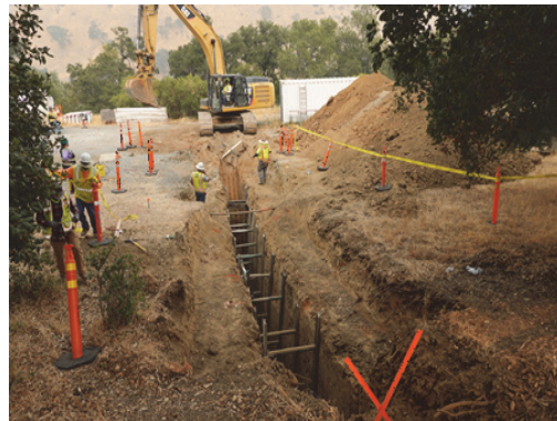
Geotech fault trenching across the site
