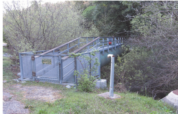
CSPL2 creek crossing
