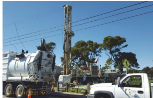
Deep Anode Installation – Corrosion Phase 1
