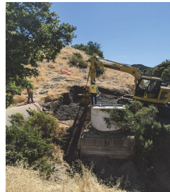
Excavation of Pipeline to Locate Source of Leak
