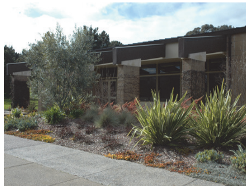
Existing Administration Building
