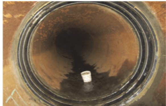
Typical Pipeline Repair with WEKO Seals
