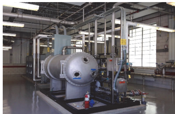
Example of Ozone Generator Unit
