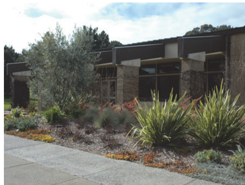
Existing Administration Building
