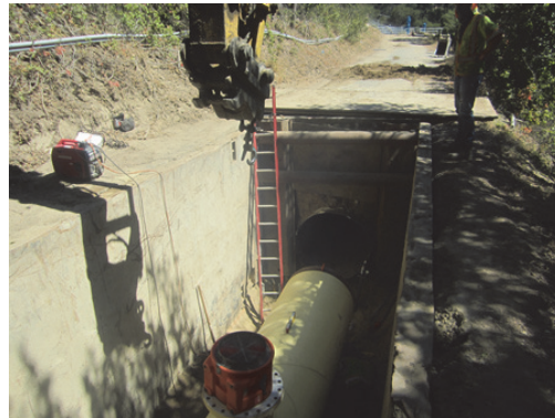
Pipeline Replacement Work inside Harry Tracy Water Treatment Plant
