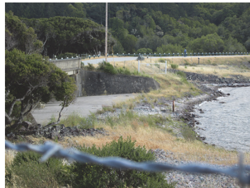
San Andreas Dam and Spillway
