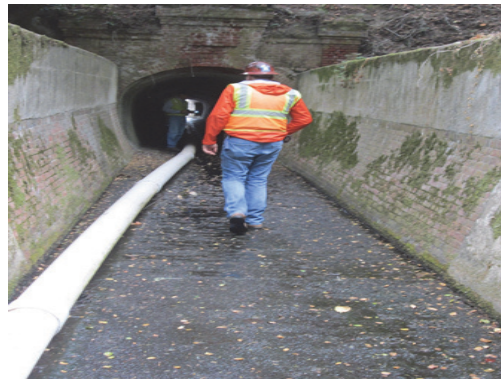
Pilarcitos spillway inspection
