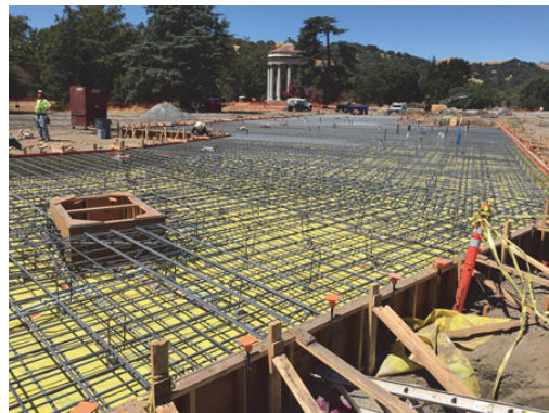
Building Slab Rebar Installation
