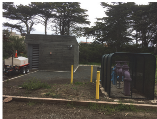
North Lake Well Station
