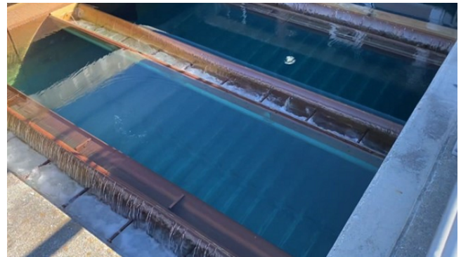
Filter Box and New Underdrain Testing
