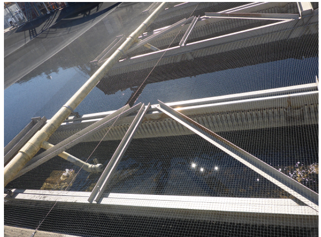
Bird Netting on Sedimentation Basin
