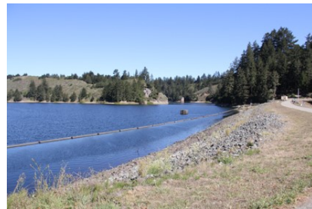
View from Pilarcitos Dam Looking Upstream
