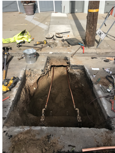
City Distribution Division Construction Staff Performing Service Line Replacement
