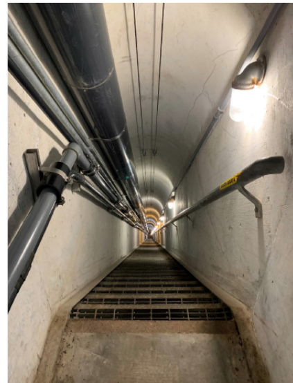
View of the Concrete Intake Shaft from the Control House
