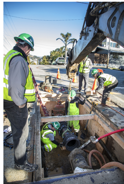
Diamond Street Water Main Replacement
