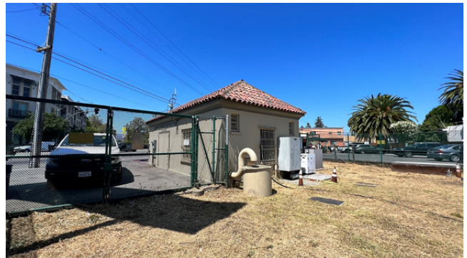
Valve Lot where New Valve will be Installed for Safe Entry
