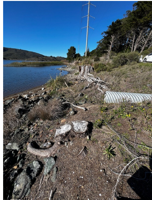
Existing San Andreas Wetlands culvert to be replaced
