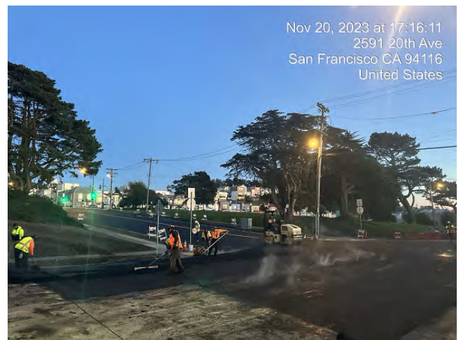
Contractor is completing the permanent paving on Vicente Street
