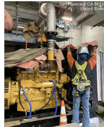
Building 821 500 kW generator exhaust system installation in December 2023.
