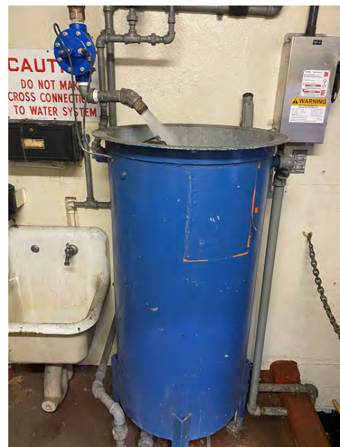
Water Connection Field Testing
