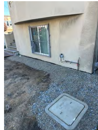
Completed Installation of a French Drain and Sump Pump
