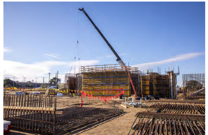
Biological Nutrient Removal (BNR) Facility Wall Placement
