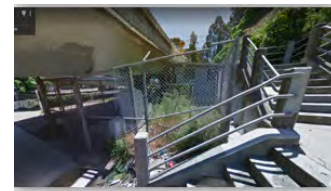
Cesar Chavez Pump Station
