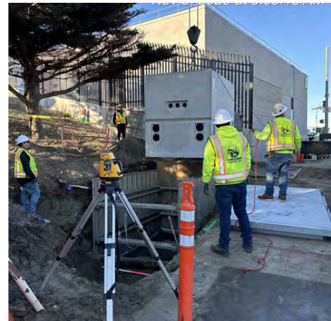
Westside PS new power service precast vault installation in November 2023.
