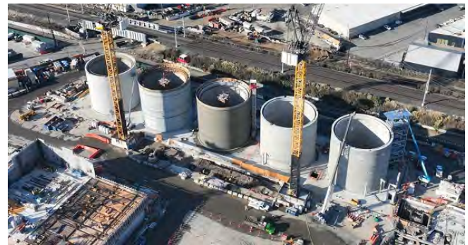
Digesters Under Construction
