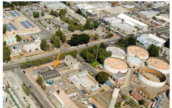
Southeast Plant- Abandoned DAF Units
