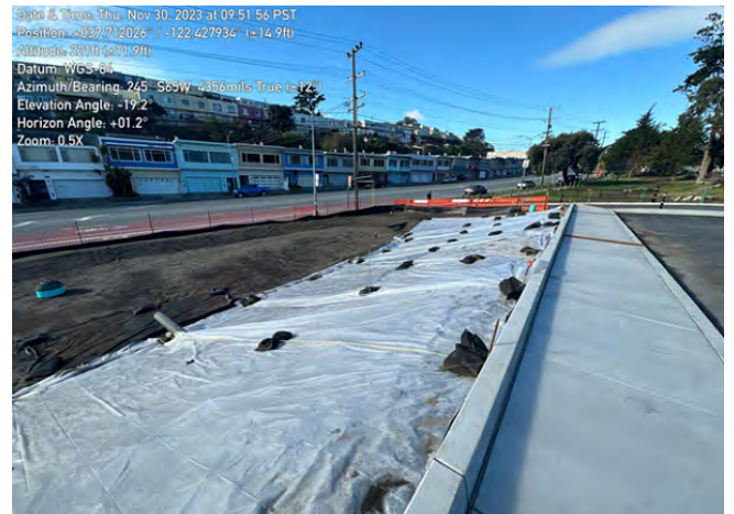
Construction of New Rain Garden at Crocker Amazon Parking Lot Entrance.
