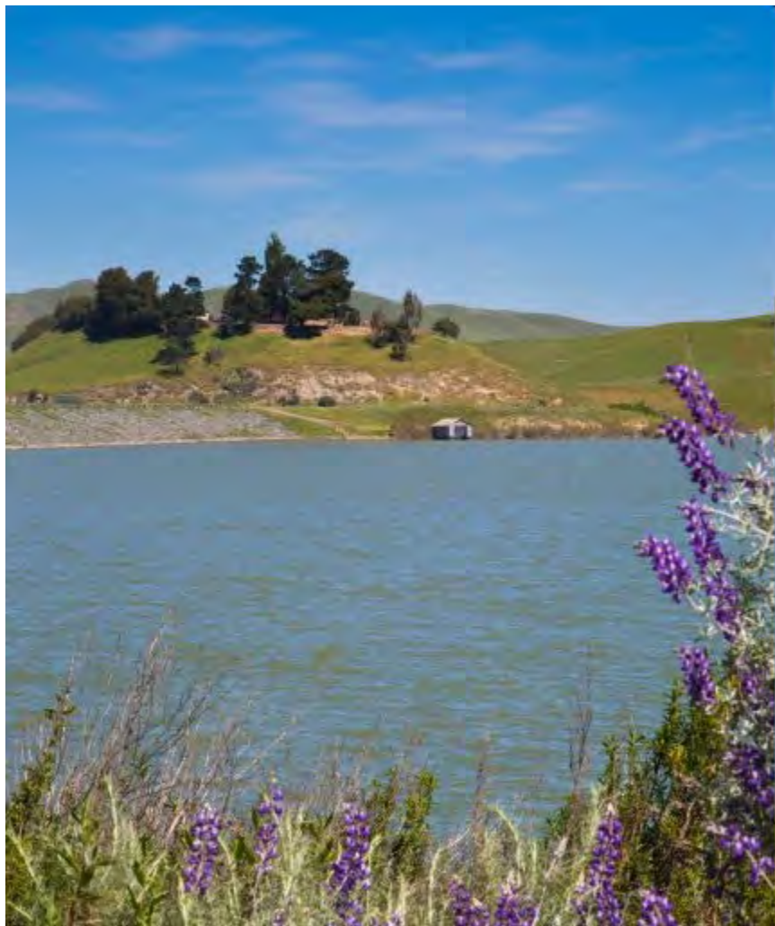
Photo: Alameda Watershed, Turner Dam at San Antonio Reservoir, April 2016
