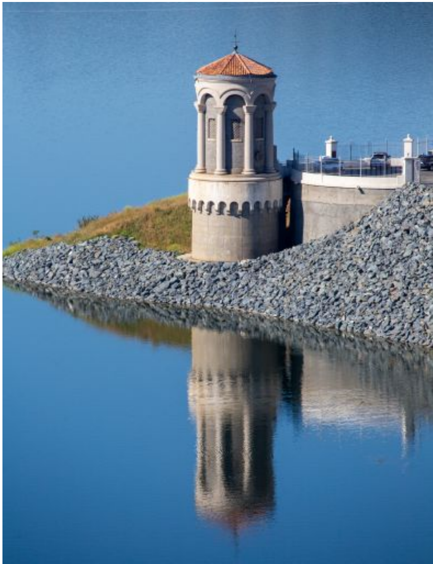
Photo: Calaveras Dam Intake Outlet Shaft Tower, June 2019
