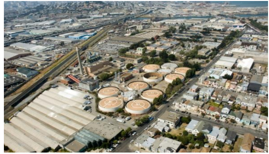
Southeast Treatment Plant
