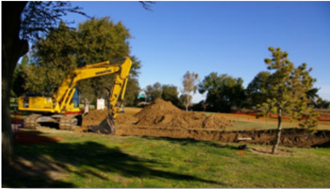
HHWP crews maintaining facilities on the ROW.
