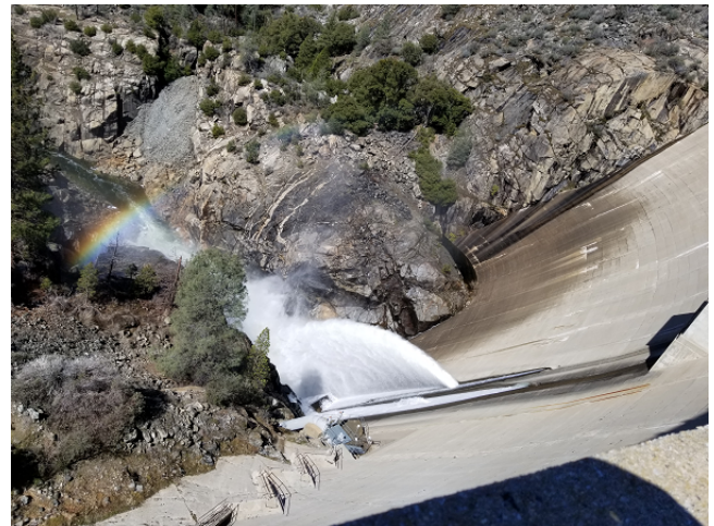
O'Shaughnessy Dam Outlet Valve Release
