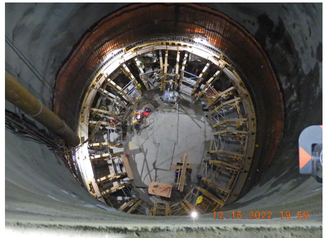
Bottom of FCF Shaft Preparing for Final Lining Concrete Pour
