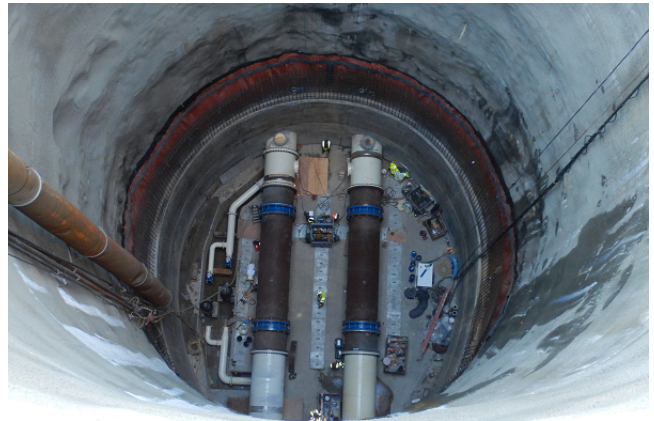
Bottom of Flow Control Facility shaft showing installed water piping
