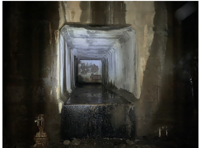
Existing condition of concrete plug
