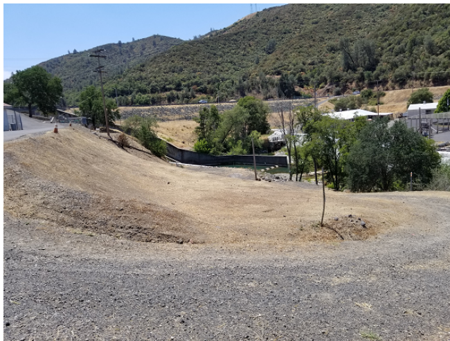
Moccasin Dam and Spillway
