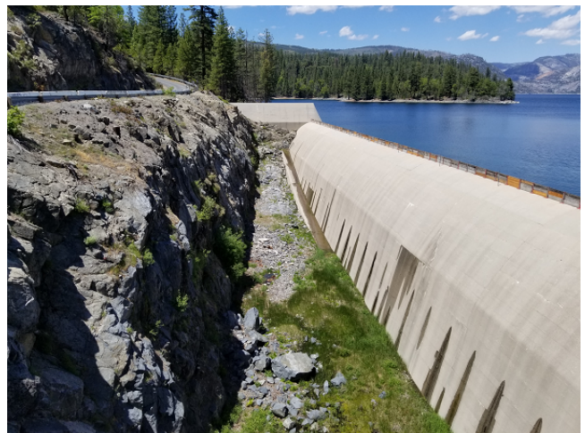
Cherry Valley Dam Spillway
