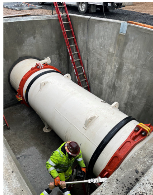
Coupler tightening of a Removable Spool Piece at Oakdale Portal [HH-1005]
