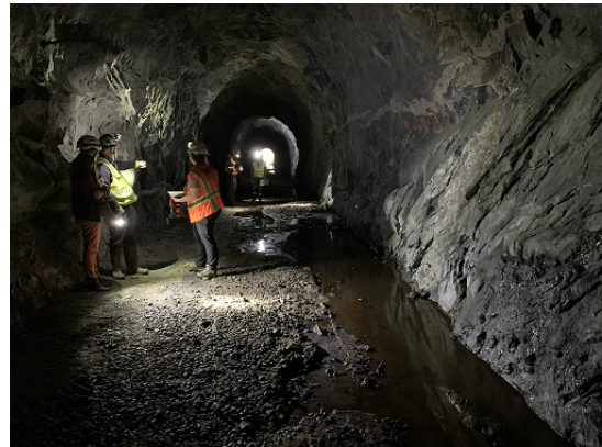
Site visit to evaluate the existing plug at Hetch Hetchy Adit within the Canyon Tunnel
