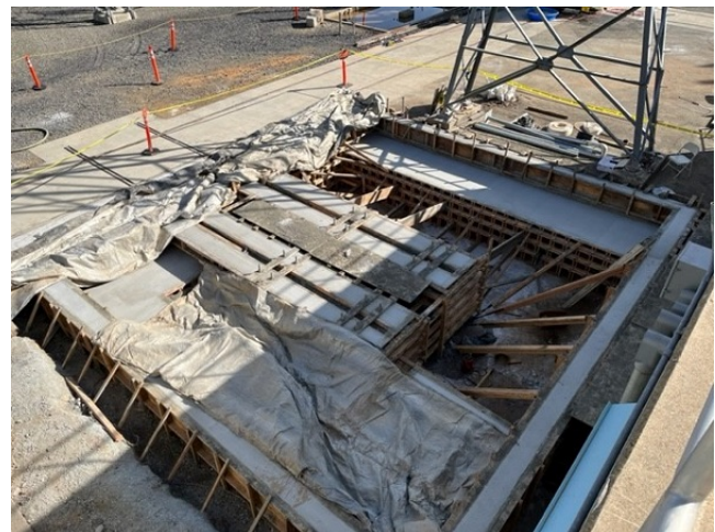
MPH HH-1003R GSU2 Foundation
