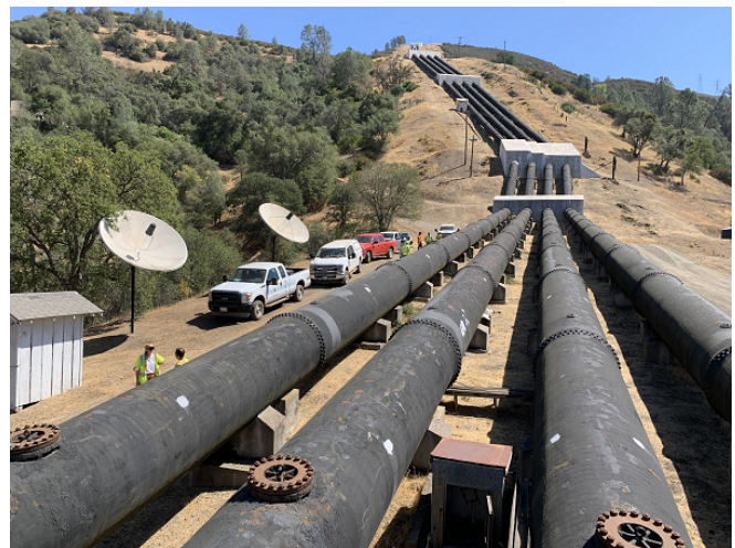
Joint Site Visit to kick off Phased Array Ultrasonic Testing effort
