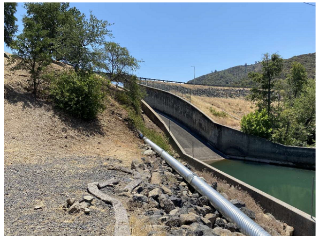
Moccasin Dam and Service Spillway
