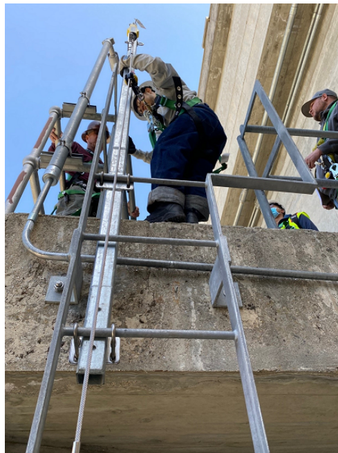
New Ladder to Spillway and Fall Protection System
