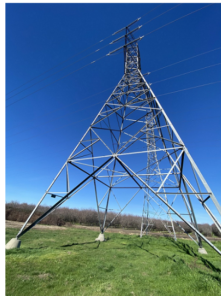
Transmission Line 7/8 Tower 508S Looking North
