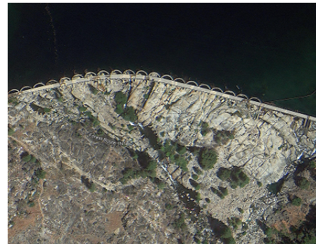
Aerial View of the Lake Eleanor Dam Bridge
