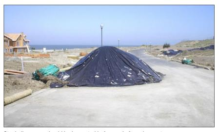
Stockpile covers should be inspected before and after rain events.
