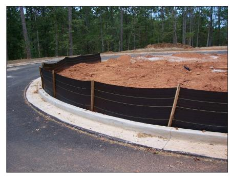
Silt fence can be used to contain sediment from disturbed areas.
