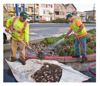
Maintenance workers remove sediment from a sediment basin in a bioretention planter on Cesar Chavez St in San Francisco. Photo: Robin Scheswohl
