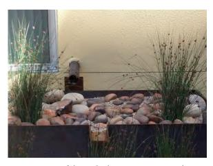
An interior roof drain discharges to a courtyard bioretention planter in San Francisco, CA. This properly designed and permitted stormwater facility is an example of an "approved alternate location" for stormwater discharge. Photo: Polly Perkins
