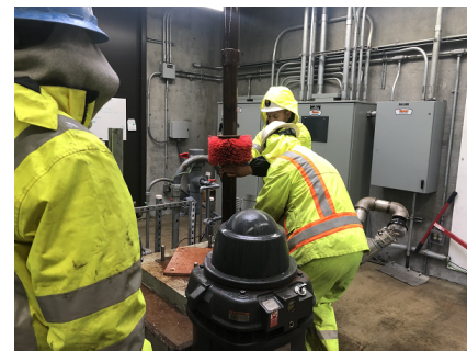
Well brushing at Colma BART Well Facility
