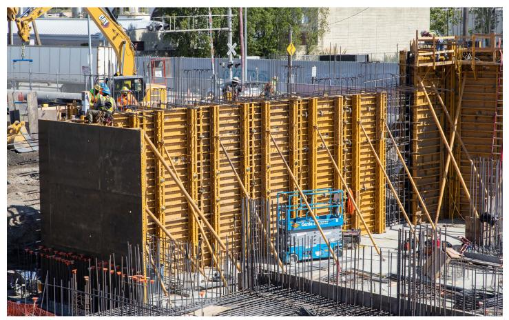
Southeast Wastewater Treatment Plant (SEP), Headworks Facility Project: Concrete pour on wall in Grit Tank Area 45.
