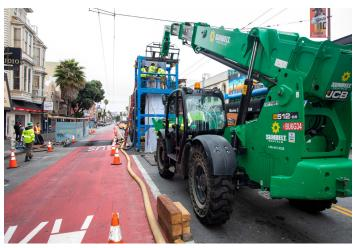
Mission Street, 16th to Cesar Chavez, Brick Sewer Rehabilitation Project: The project uses a trenchless method called cured-in-place pipe (CIPP) technology to rehabilitate the brick sewer tunnel.
