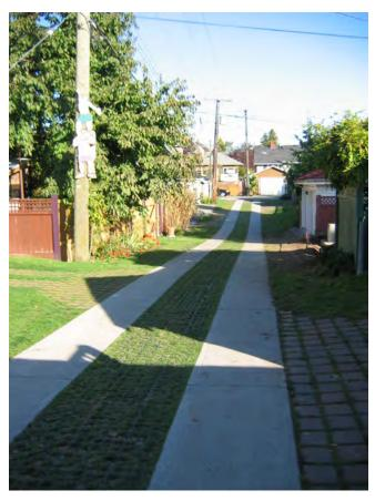
"Country Lanes" in Vancouver, Brtitish Columbia enhance the alley's aesthetic quality and reduce stormwater discharge to the City's stormsewer system by allowing runoff to flow over vegetation and infiltrate into the ground. Photo: Rosey Jencks
