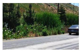
This vegetated buffer strip along the Imperial Highway in Los Angeles, CA slows stormwater runoff from the highway. Photo: LA Stormwater Program
