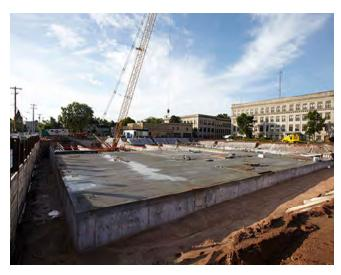
Construction of an underground stormwater detention basin beneath the City Hall parking lot in downtown Oshkosh, Wisconsin. Photo: Precast-Prestressed Concrete Institute
