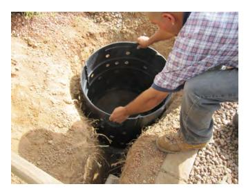
Installation of a pre-cast drywell, note the holes to allow stormwater infiltration. Photo: Lake George Association
