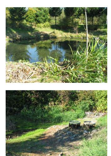
An infiltration basin in Waterworks Gardens at the King County East Division Reclamation Plant, Renton, WA, is part of an environmental art park that treats stormwater. Runoff flows through stormwater treatment ponds, and the wetlands form an earth/water sculpture that funnels, captures and releases water. Photo: Rosey Jencks
