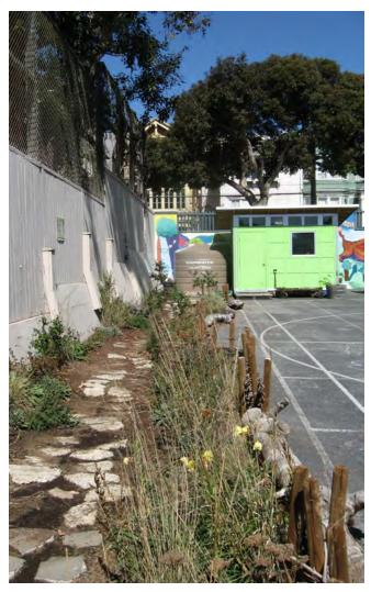
The rainwater harvesting system at New Traditions Elementary School in San Francisco, CA overflows to a vegetated area before flowing into the sewer system. Photo: Polly Perkins
