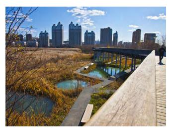
Constructed wetlands not only create a park-like settings, but they also remove contaminants from stormwater and provide flood control. Photo: Programmed Property Services
