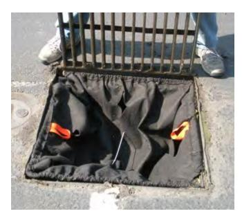
Drain insert in a stomrwater catch basin. Photo: EnviroMet
