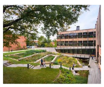
This project's constructed wetland treats the building's wastewater on-site while the pond and rain garden prevent stormwater runoff. Photo: Albert Vecerka
