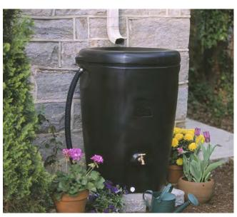
A disconnected downspout and rain barrel. Photo: Clean Air Gardening
