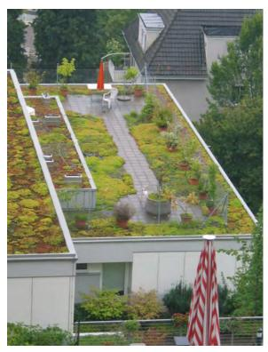
Intensive vegetated roofs can provide usable open space in addition to their stormwater management function. Photo: Rosey Jencks
