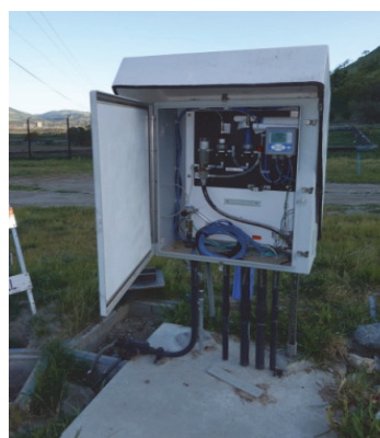
Sunshade installed for the water quality equipment
