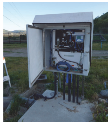
Sunshade installed for the water quality equipment
