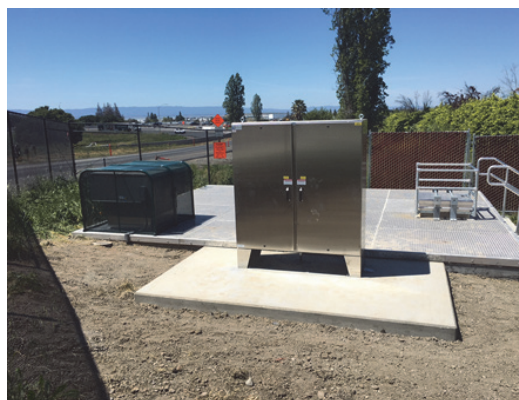
Ventilation and Sump Pump Project
