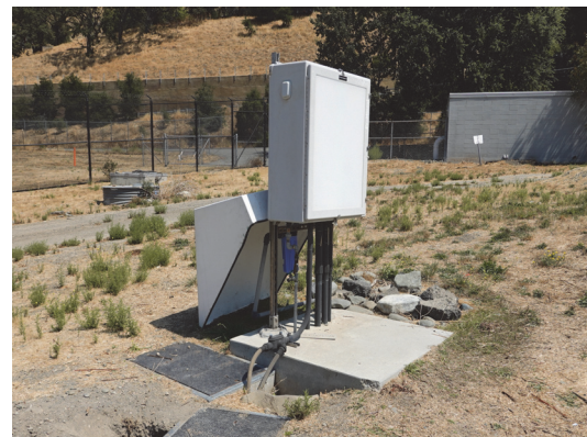
Sunshade and Pressure Relief Valve to be installed at the SABPL Chemical Analyzer Cabinet
