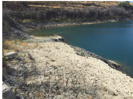
Current Condition of Pond F2 Access Road
