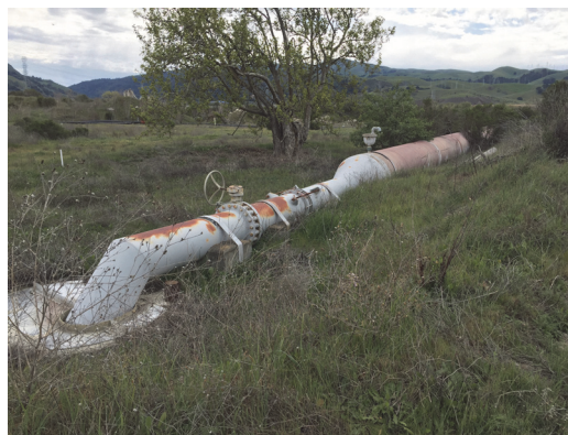
Existing Aboveground Pipe to be Demolished
