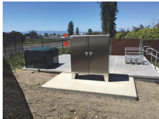
Ventilation and Sump Pump Project
