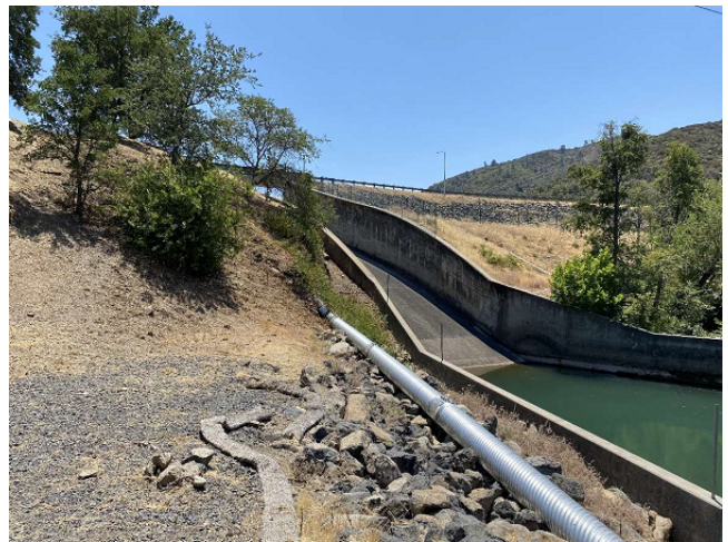
Moccasin Dam and Service Spillway
