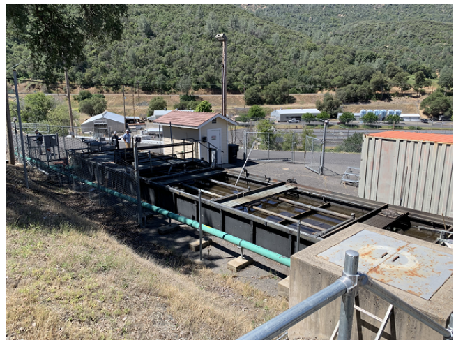
Existing condition of Moccasin Wastewater treatment plant
