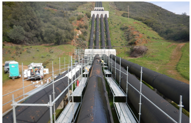
Coating of exposed pipes upon completion of Phased Array Ultrasonic Testing
