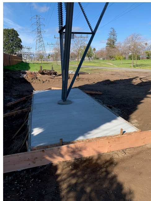
Completed concrete foundation at Structure 608 [HH-1007]
