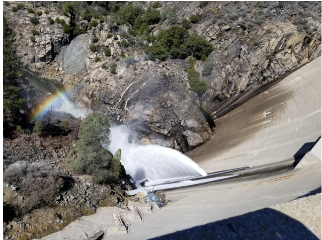
O'Shaughnessy Dam Outlet Valve Release
