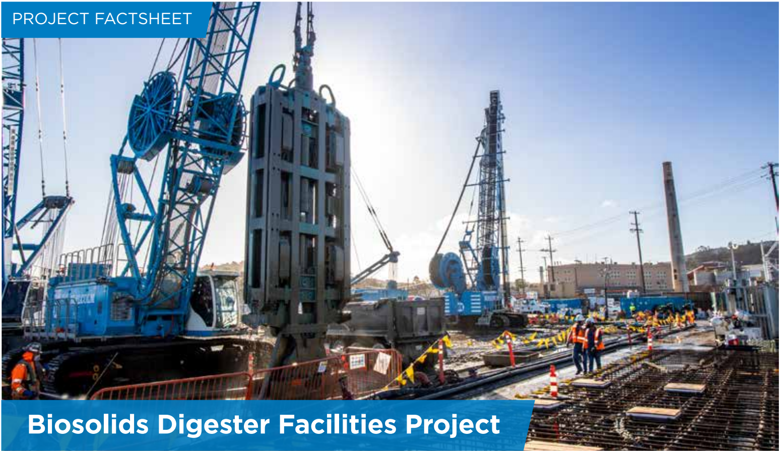
Pictured above: Biosolids Digester Facilities Project Construction
