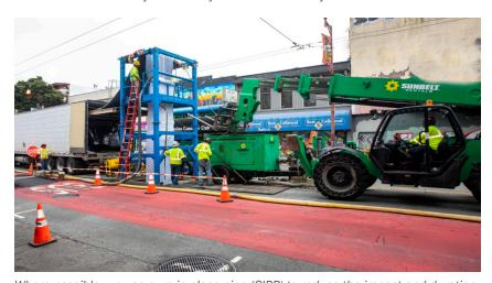
Where possible, we use cure-in-place-pipe (CIPP) to reduce the impact and duration of our work in the street. This method can often reduce the duration of work.
