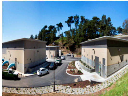
Completed Lake Merced Pump Station Buildings
