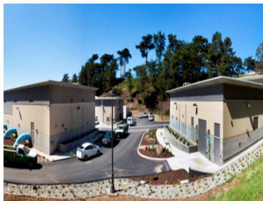
Completed Lake Merced Pump Station Buildings
