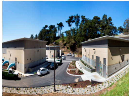
Completed Lake Merced Pump Station Buildings
