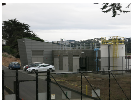
Lake Merced Well Station
