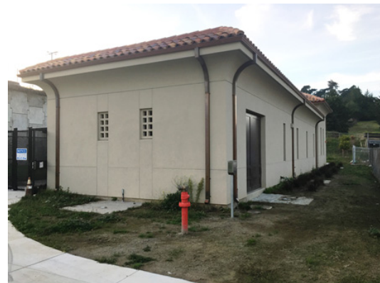
Exterior of completed Serramonte Blvd well station in Colma, undergoing testing.
