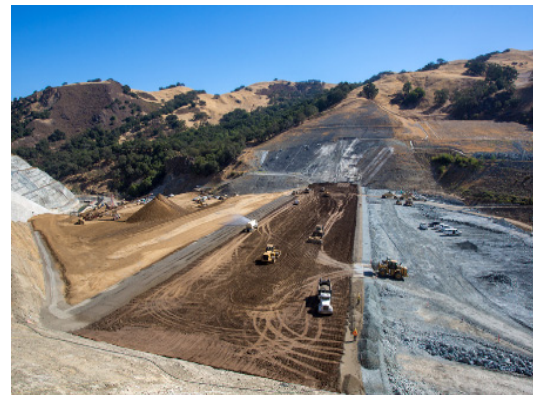
Placement of Dam Embankment
