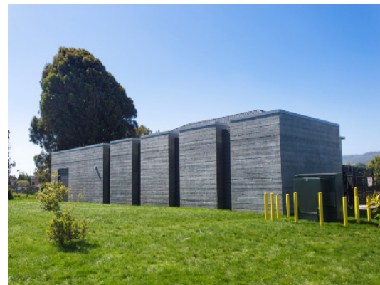
Exterior of completed Linear Park well station, undergoing testing
