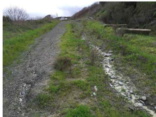
Existing Access Road to Pond F2
