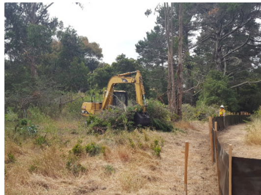
WD-2654R: Adobe Gulch Site with erosion control and flags to mark acorn planting locations
