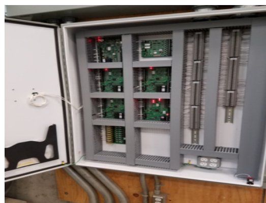
Security Panel recently installed
