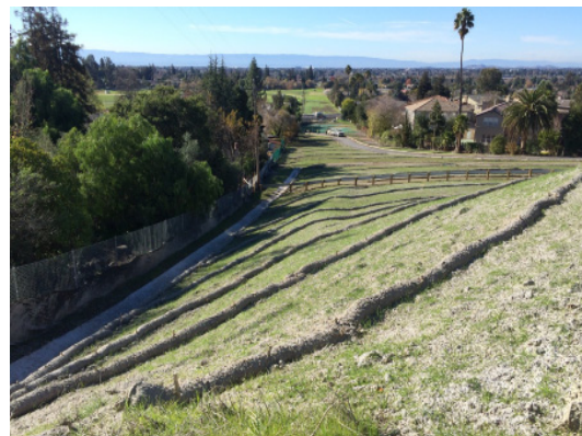
Site restoration was completed at Irvington Portal staging area
