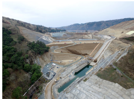
Progress made for the Dam Embankment in 2017
