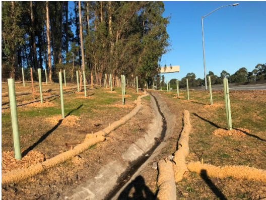
LCSD Oak Tree Planting within Caltrans ROW
