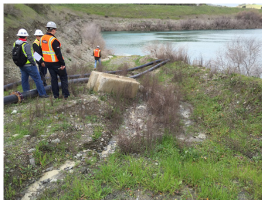
Existing Access Road to Pond F2
