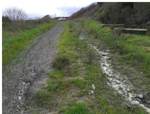
Existing Access Road to Pond F2
