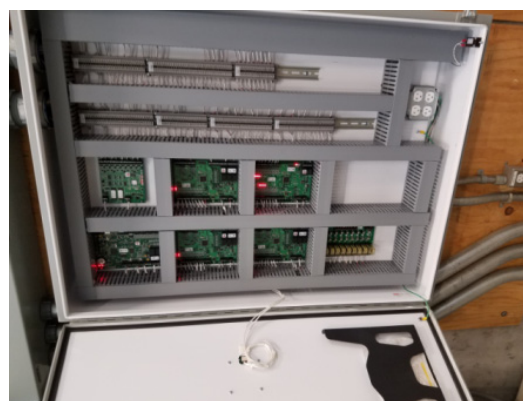
Security Panel recently installed
