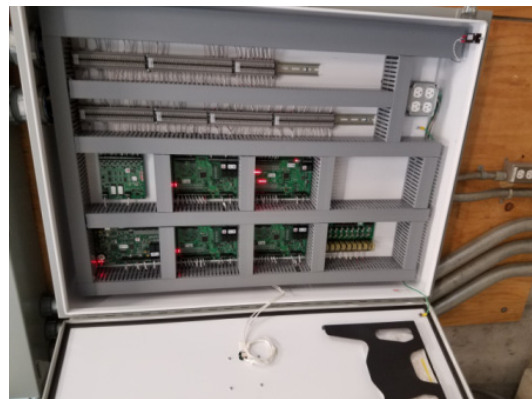
Security Panel recently installed
