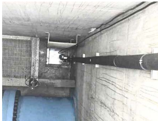
Sump pump installation inside of vault 4
