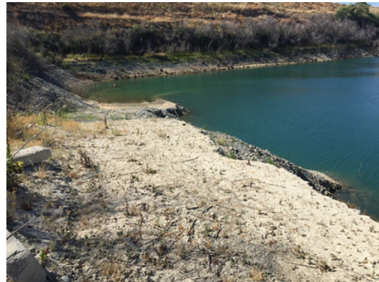
Current Condition of Pond F2 Access Road
