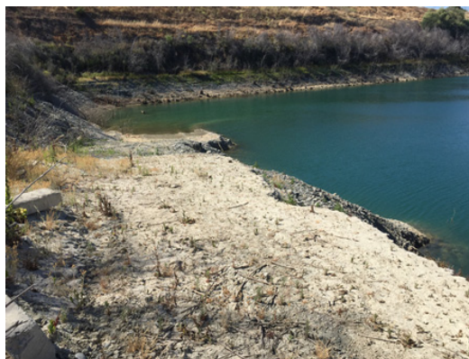
Current Condition of Pond F2 Access Road
