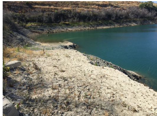
Current Condition of Pond F2 Access Road
