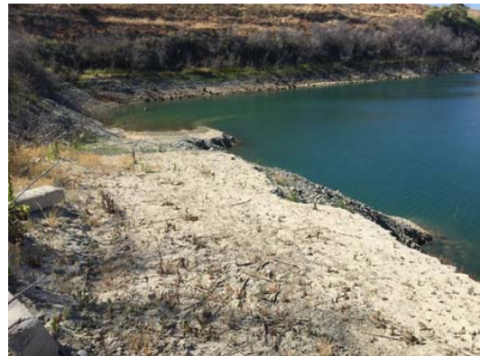
Current Condition of Pond F2 Access Road
