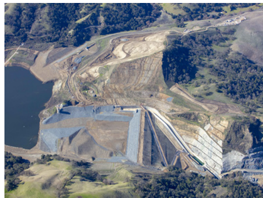
Completion of the Approach Channel
