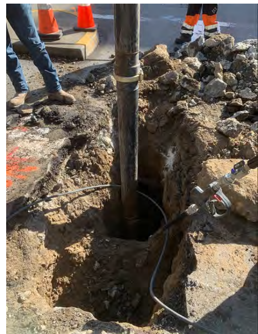
PG&E Pothole Investigation at 6th and Geary
