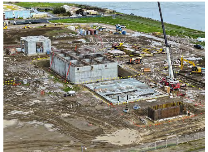
New Treasure Island Treatment Plant Aerial View of General Job Site
