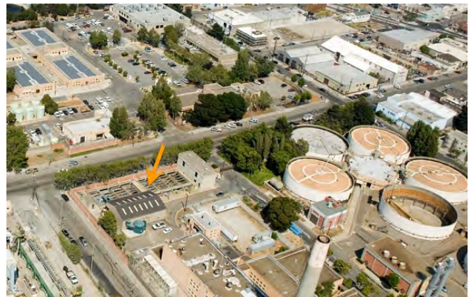
Southeast Plant- Abandoned DAF Units
