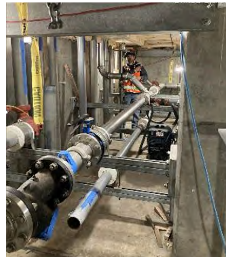
OSP Building 800 Utility Trench
