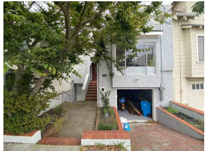
118 Noriega Street Floodwater Grant Project - Before Construction
