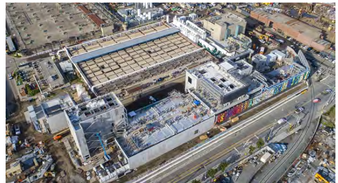
New Headworks Facility Aerial View Looking South
