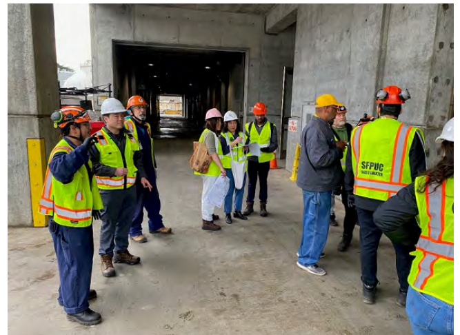
The Project Design Team Completed Field Walk-Thru with Operations, Engineering and Maintenance Staff
