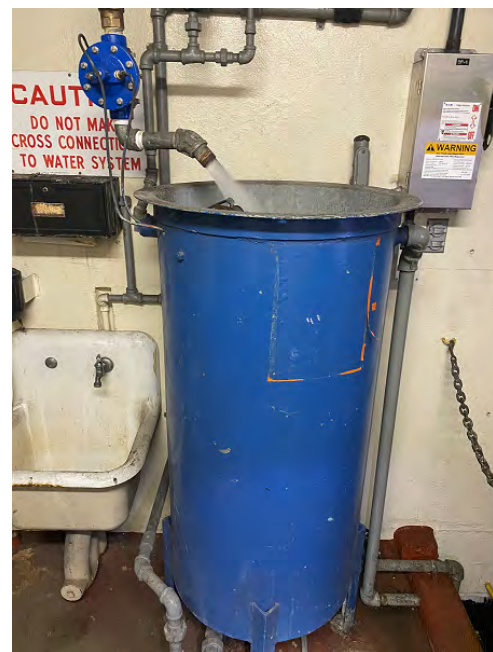
Water Connection Field Testing
