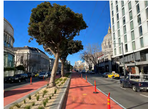
Sewer Completion along Van Ness Avenue
