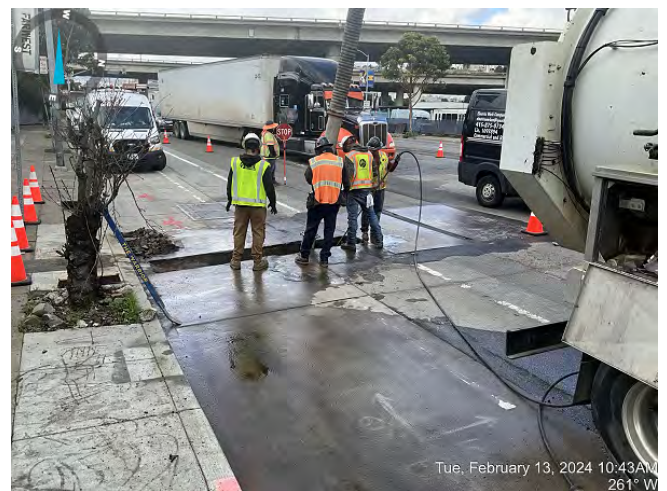
Contract A: Slot Trench Vacuum Excavation for Utility Location
