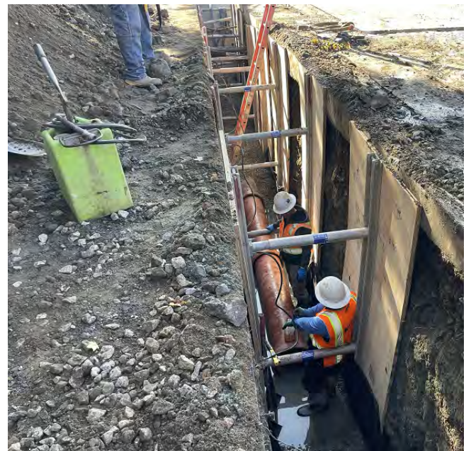
Installation of Combined Sewer on 15th Street
