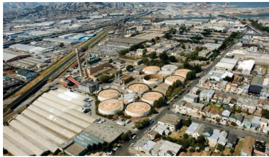
Southeast Treatment Plant
