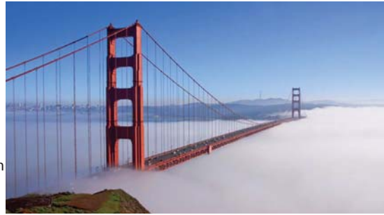
Fog on Golden Gate Bridge
