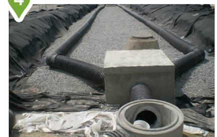
An underground stormwater storage structure filled with gravel that receives runoff through horizontal pipes below the pavement surface. This project includes over 10,347 square feet of infiltration gallery to help store stormwater and slowly release it into the groundwater aquifer.
