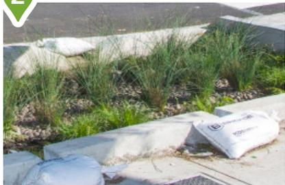
Rain gardens capture stormwater runoff from streets, roofs, and parking lots. Plants and soil absorb that water, reducing the amount of runoff entering the sewer system. This project has constructed a total of 32 rain gardens covering 6,746 square feet between Lands End Trail Eagle Point and the California Coastal Trail entrance at 25th Ave North.
