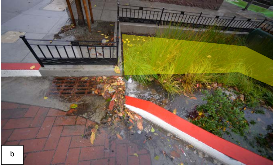
Figure 11 a and b: (a) Schematic section of a typical Oak & Fell bioretention bulbout, (b) the Broderick St SW bulbout during a very large storm event in Dec 2015
