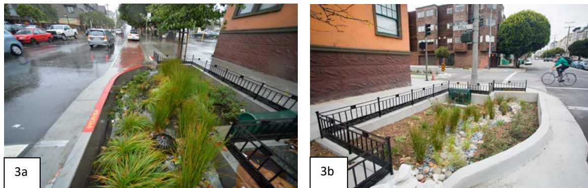
Figure 3a and 3b: The bioretention bulbout planter and permeable paving on the Broderick St SW (a) from the northern perspective, and (b) from the western perspective
