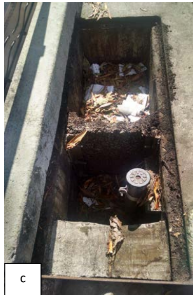
Figure 10a, b, and c: Inlet structure of Oak & Fell bulbouts (a) construction drawing, (b) clogged with debris during a storm event, and (c) with debris in dry conditions.
