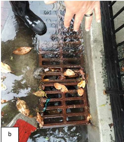
Figure 10a, b, and c: Inlet structure of Oak & Fell bulbouts (a) construction drawing, (b) clogged with debris during a storm event, and (c) with debris in dry conditions.
