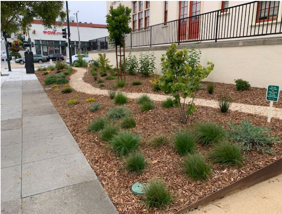
Construction of stormwater swale
