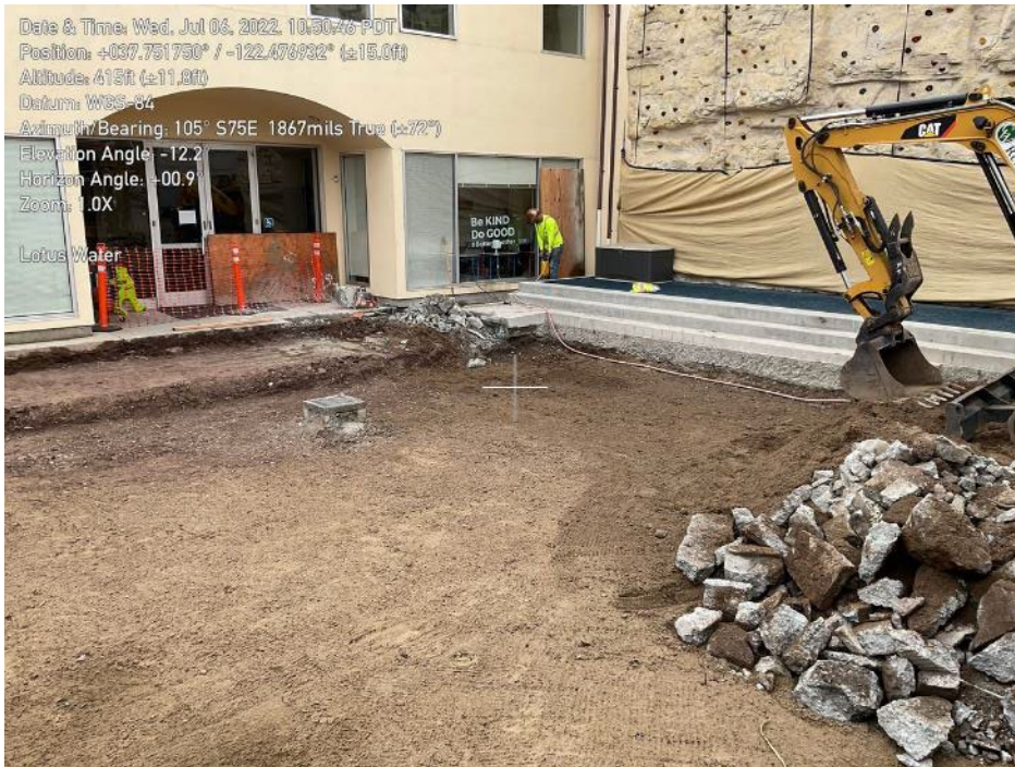
Construction of permeable pavement.
