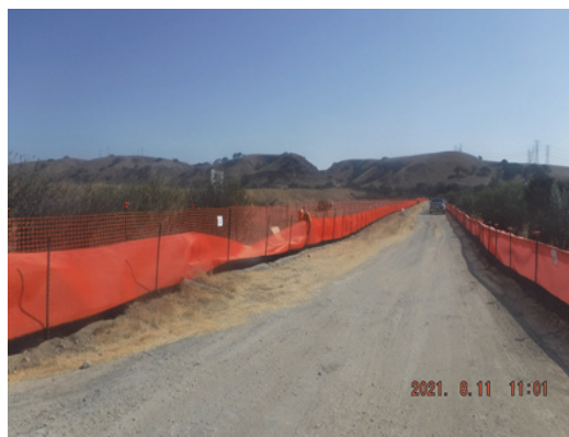
Installation of Wildlife Exclusion Fence
