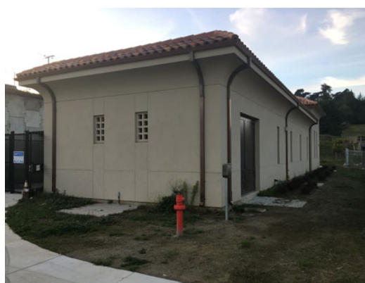
View of Poncetta Drive Well & Treatment Facility in Daly City (formerly named Lake Merced Golf Club Well Station)
