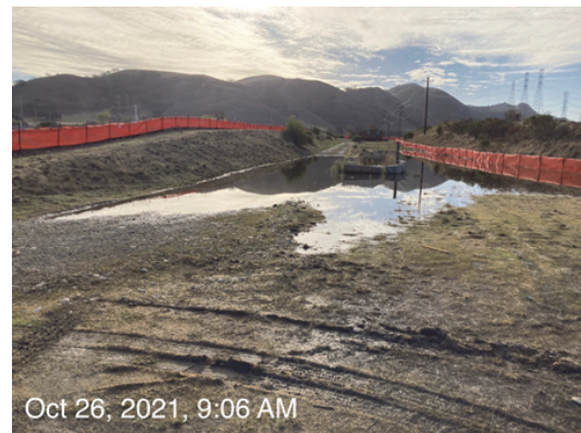
Flooding of Access Road
