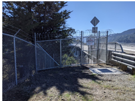
Fence and gate towards the entrance into the Lower Crystal Springs Dam at the northside
