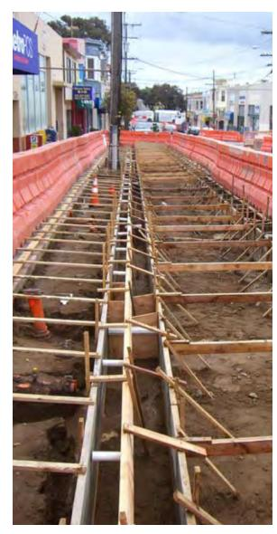
Leland Avenue, San Francisco, under construction. Permeable pavement will be installed on the sidewalk and in the parking lane.
