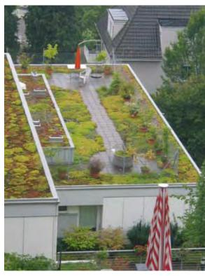
Intensive vegetated roofs provide usable open space in addition to their stormwater management function.
