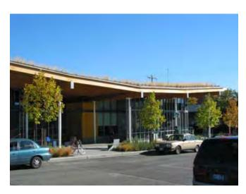
Vegetated roofs can be designed to be visible from the street to add unique textures and colors to building design.
