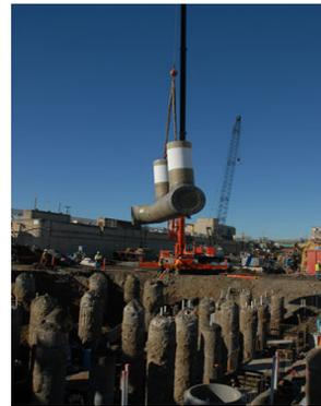
Scope III - Main Headworks, grit handling odor duct under the slab installation
