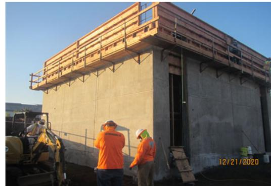
*WW-667 Forming For Parapet Wall and Trenching for Yard Piping.*
