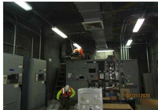
WW-651: Switchgear work during PG&E shutdown
