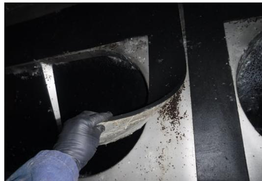
*Baker St. CSD damaged backflow preventer valve*
