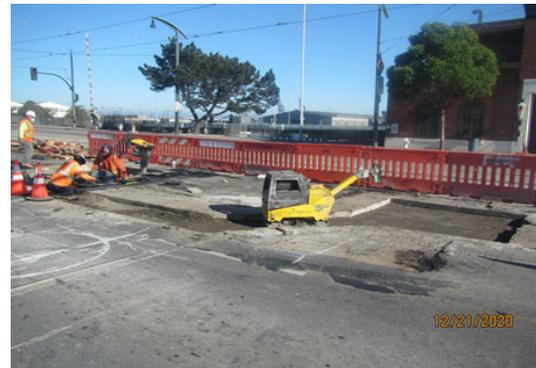
*WW-696 Backfill After 12-inch Water Line Relocation on 3rd St.*
