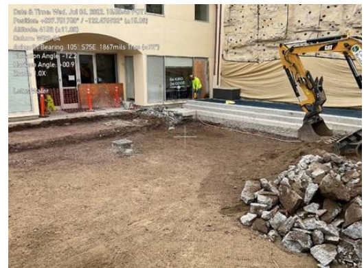
Construction of permeable concrete at Lycee Francais de San Francisco School
