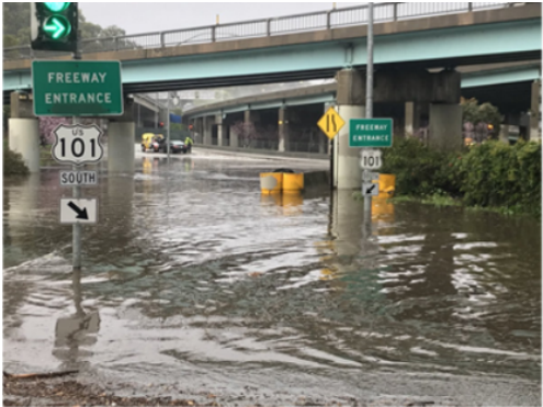
Flooding at the I-280/Hwy 101 interchange at Lower Alemany area, during the rainfall of February 13, 2019
