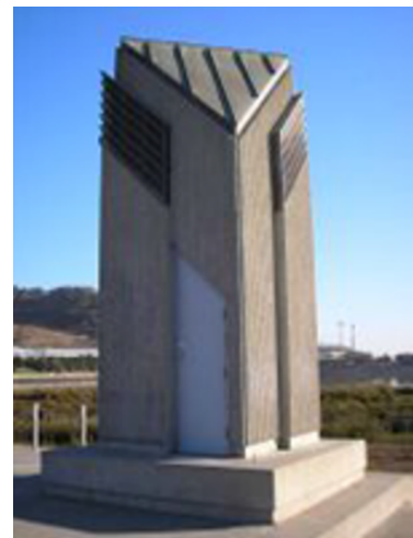
Sunnydale Pump Station
