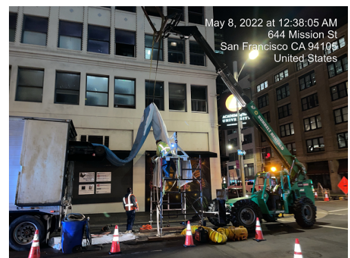
WW-712: Cured-In-Place Liner Installation on New Montgomery St
