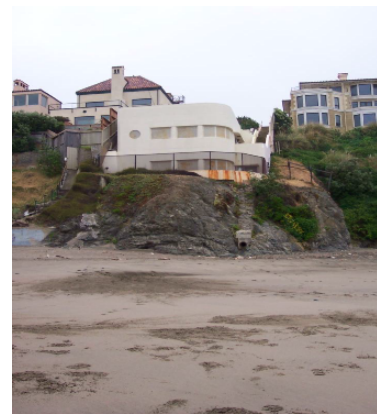
Seacliff No. 2 Pump Station and the CSD 007 discharge location at Baker Beach
