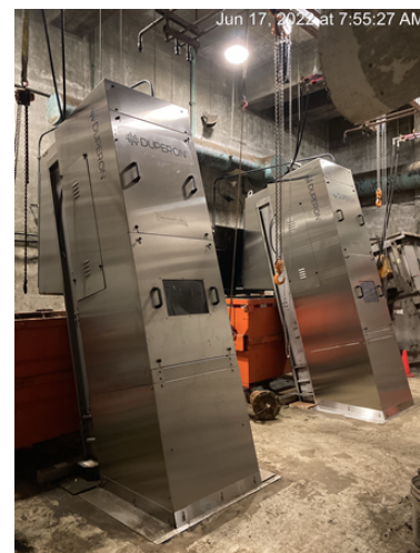
Completed bar screens in operation
