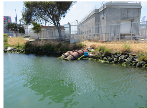
Current pipeline crossing at Islais Creek
