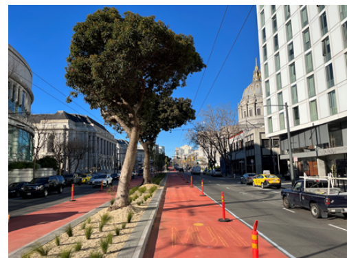
Sewer Completion along Van Ness
