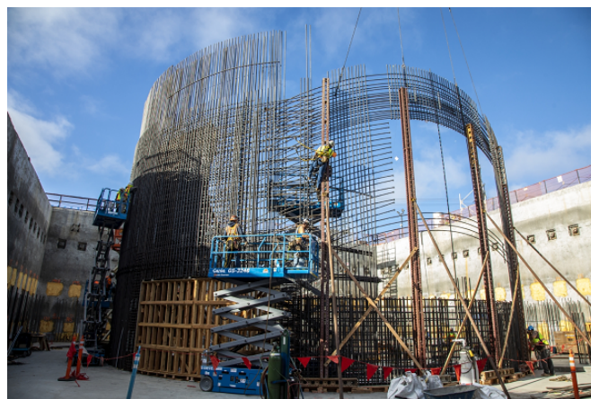
Erection of the Digester Skirt Walls
