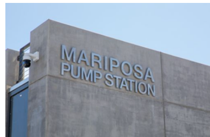
Signage Installation at Mariposa Pump Station
