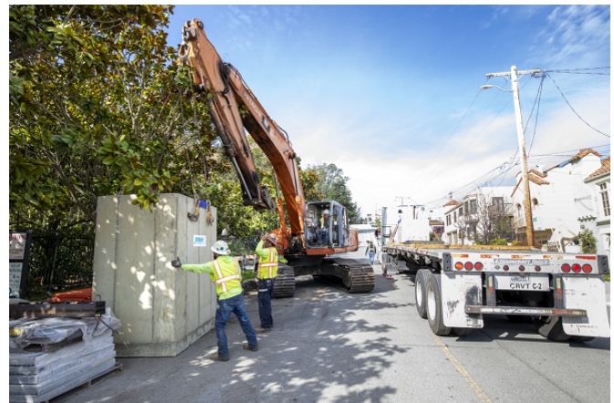
Preparing to install storm drains at 15th and Wawona
