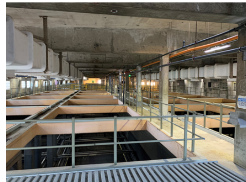
Existing SEP-041 wet-weather primary sedimentation building.
