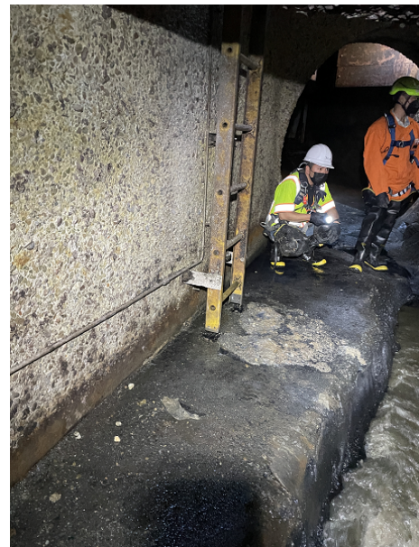
Howard CSD inspection after cleaning.
