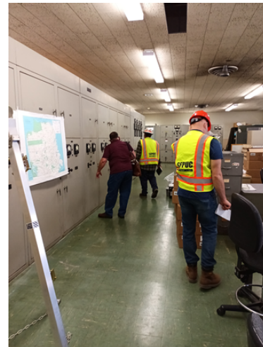
WWE staff and design team surveying existing obsolete electrical equipment at NPF 930 Administration Building.
