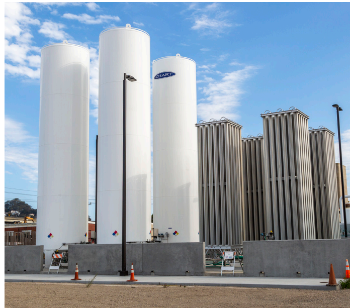
SEP Cryogenic Oxygen Generation Plant Demolition & Liquid Oxygen Upgrades
