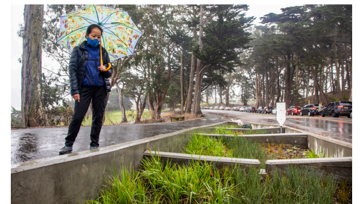
Baker Beach Green Streets: Rain gardens during wet weather on El Camino Del Mar
