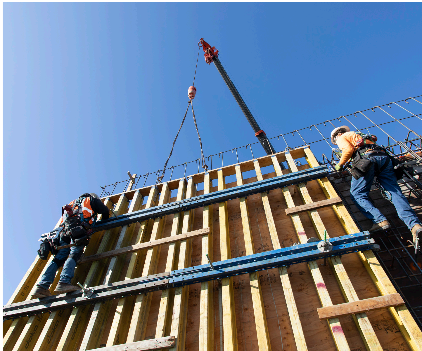
Mariposa Pump Station Improvements Project: Installing wall formwork on pump station.
