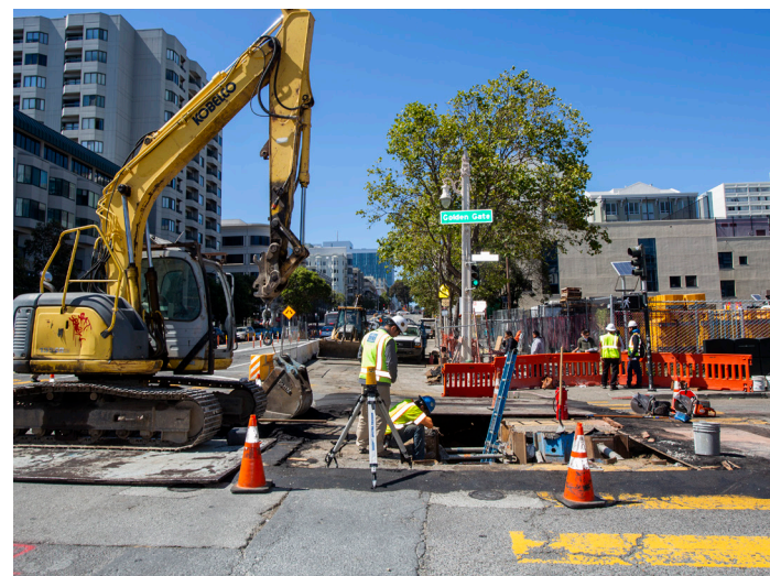
Van Ness Improvement Project: construction activity
