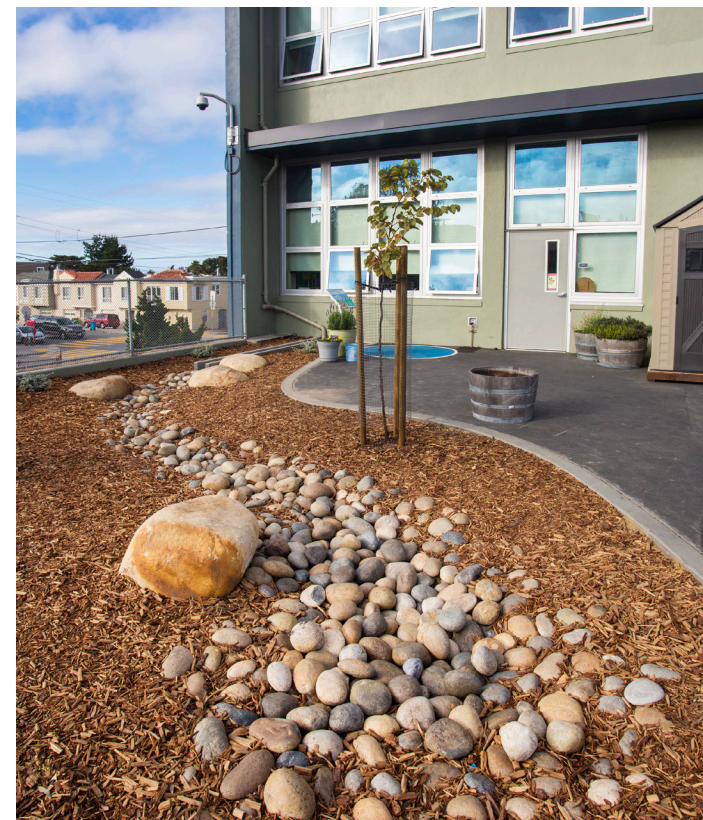
Robert Louis Stevenson Elementary School Stormwater Management Project, green infrastructure grant awardee
