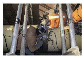
Installation of a New 36-inch (36") Diameter Welded Steel Pipe (WSP) at 19th Avenue and Sloat Boulevard
