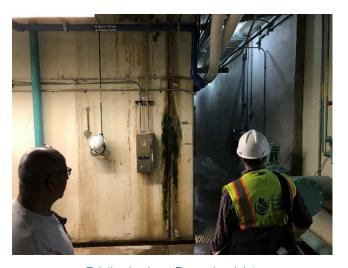
Existing Leaks at Expansion Joints
