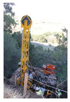
Geotechnical Boring performed by Helicopter Access
