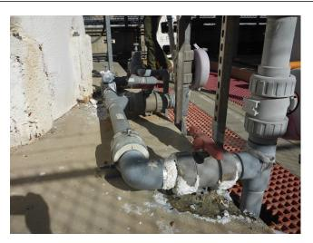
Concrete Damage at Caustic Soda Line
