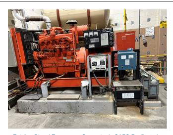
Existing Diesel Emergency Generator in SAPS Facility to be Replaced with New Propane Generator for Backup Power
