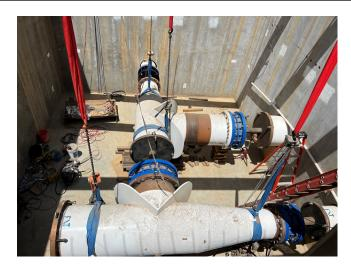
Inside of Valve Vault with recently installed Valve Manifold Piping
